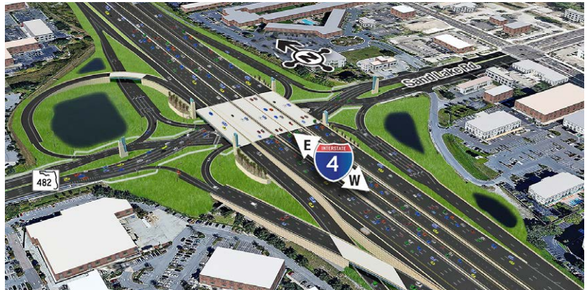
The design for this project is ongoing. The final configuration of the interchange will be similar to what is shown in this rendering, but small refinements are anticipated.
