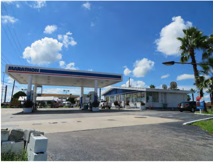
8PO07962_a Facing Southwest
