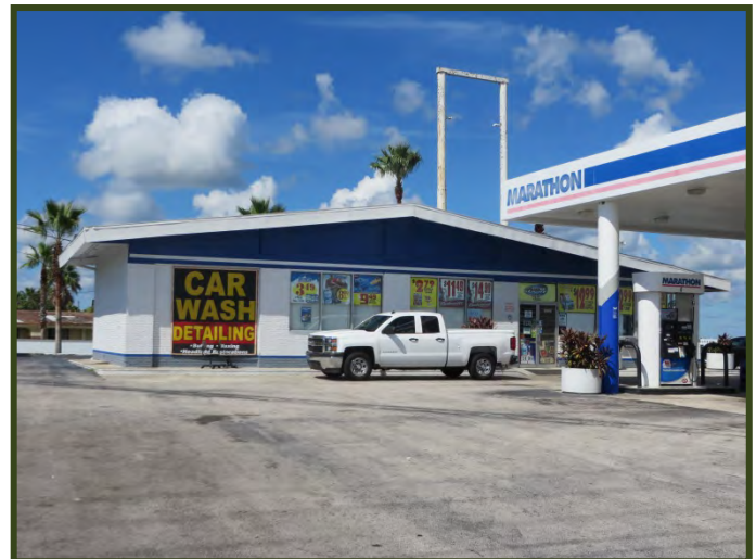
Figure 17 – Resource 8PO07962, facing west.
