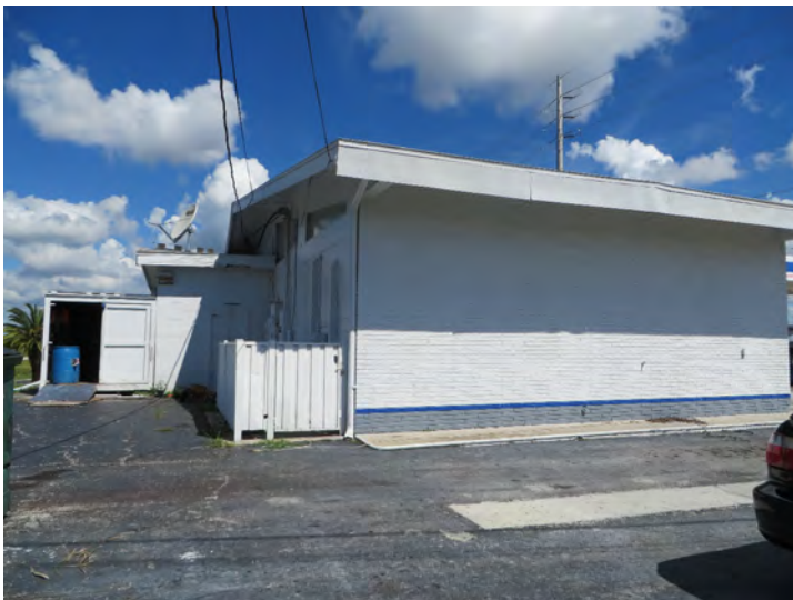
8PO07962_e Facing North
