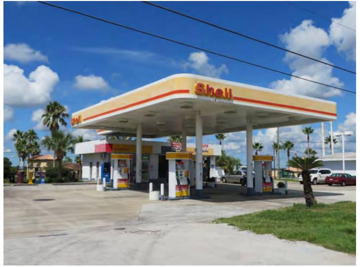
8PO07963_b Facing Northwest
