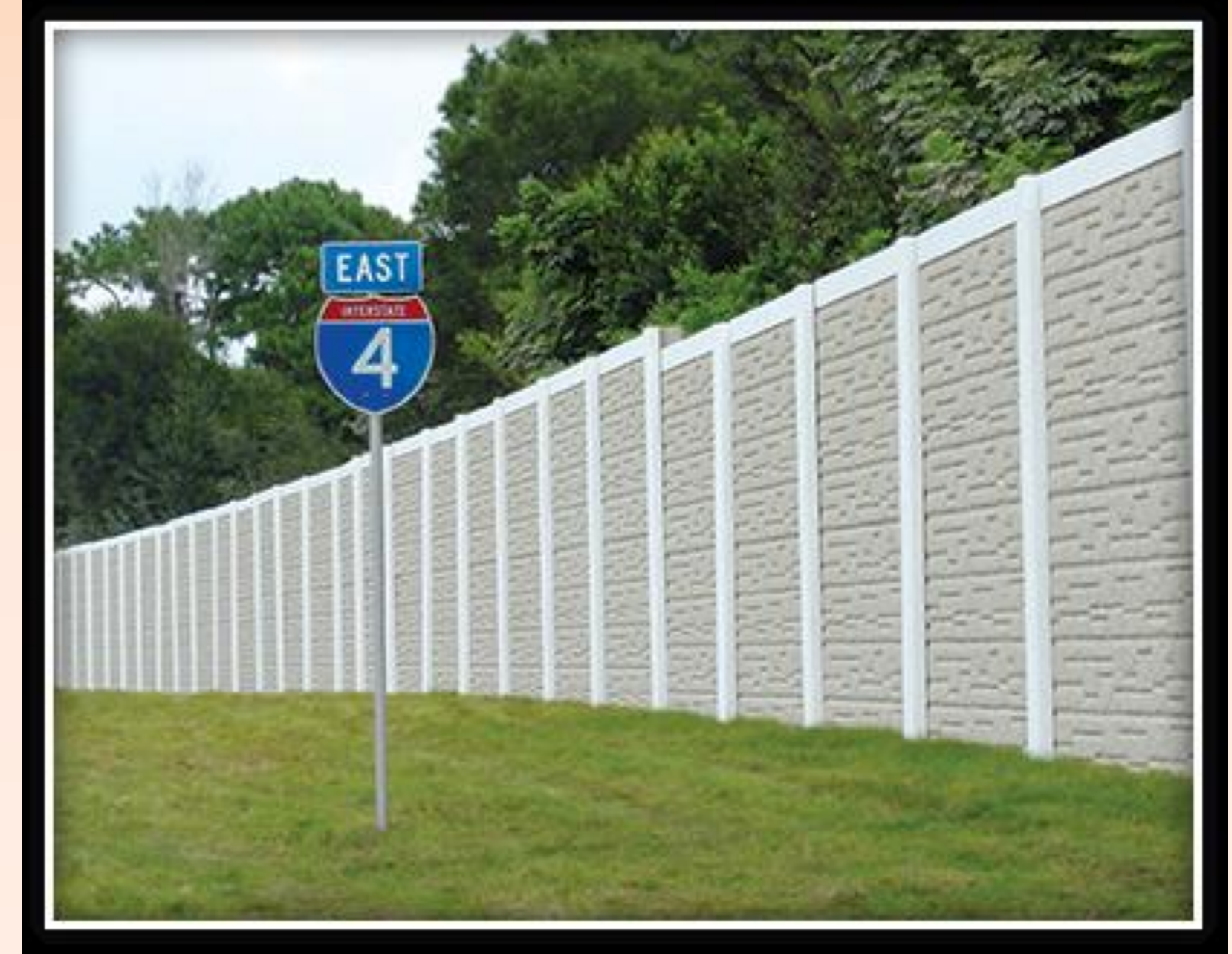
Existing Noise Barrier along I-4
