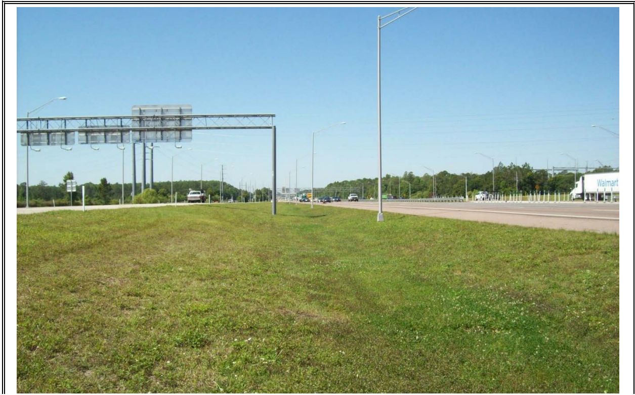
Site 16: Patco Montgomery Spill Site
