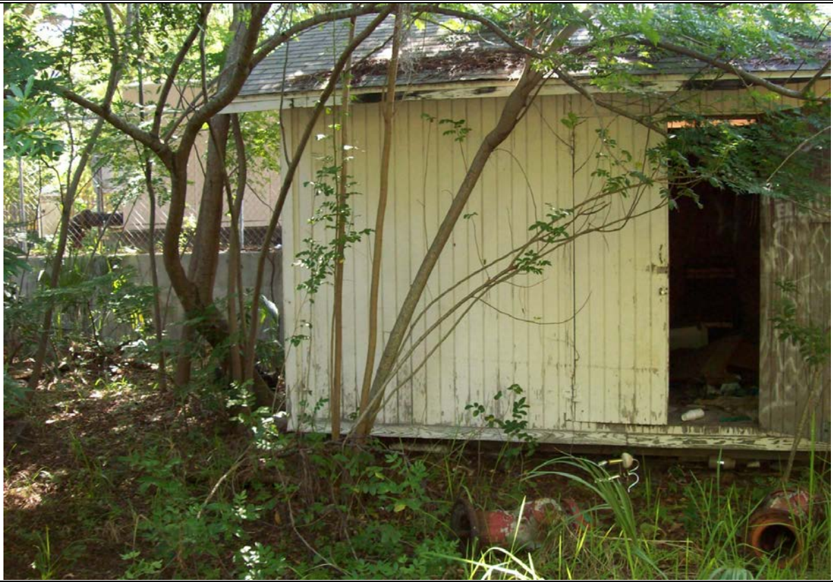
Pond Site 136B: Abandoned structure
