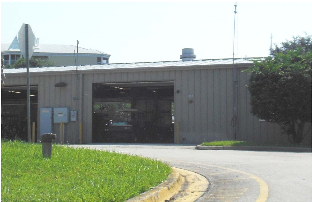
Site 76: Marriott Cyprus Pines Golf Course Maintenance Facility
