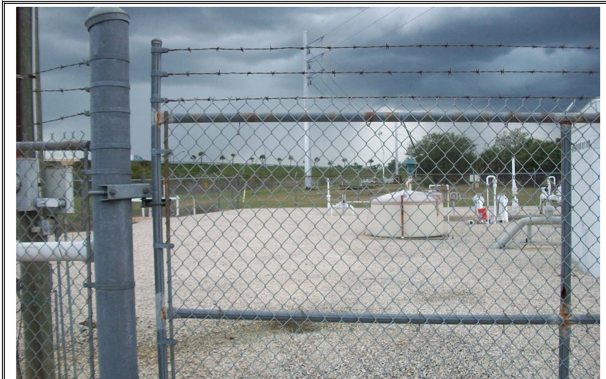
Site 10: Florida Gas Transmission Company – western facility
