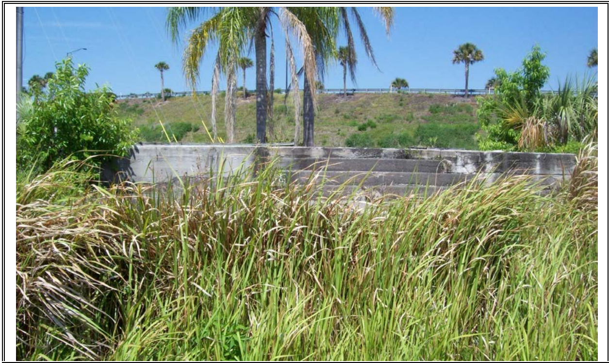
Site 10: Florida Gas Transmission Company – historic foundation
