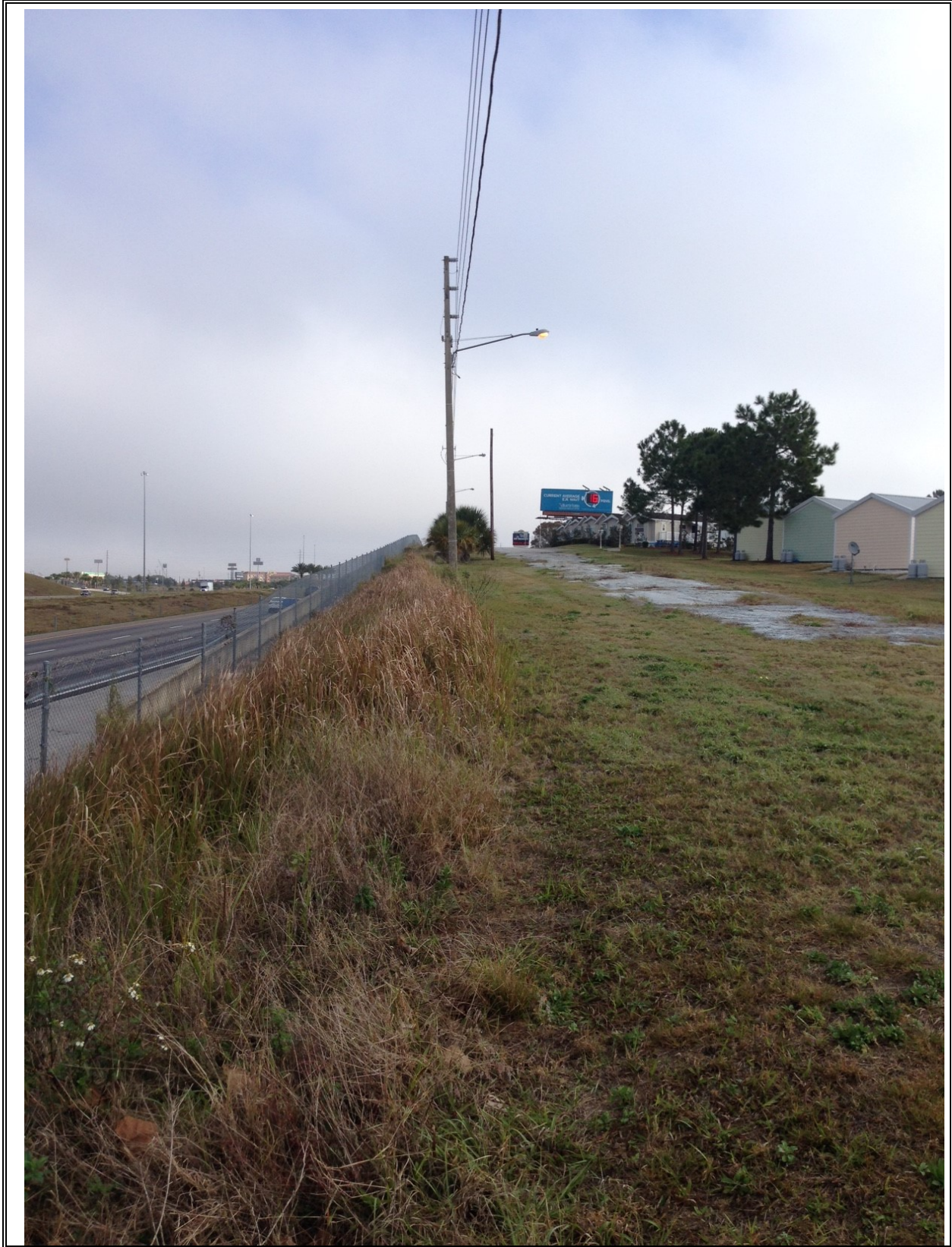
NSA A – ROW and Power Line
