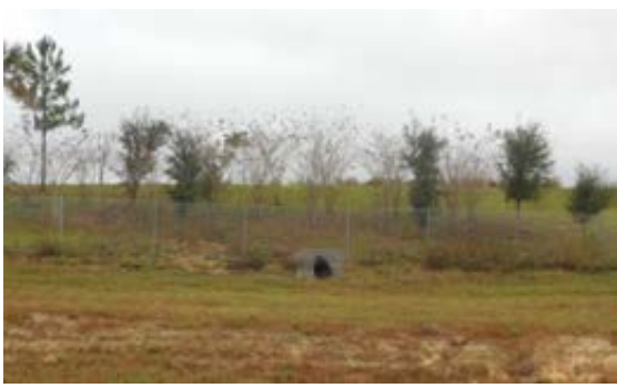
Emergency outfall from Ritchie Brothers Pond 4 to FDOT Right-of-way
