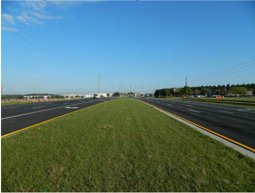
Looking N in the median of US 27, just south of the Cracker Barrel driveway, south of Dunson Road
