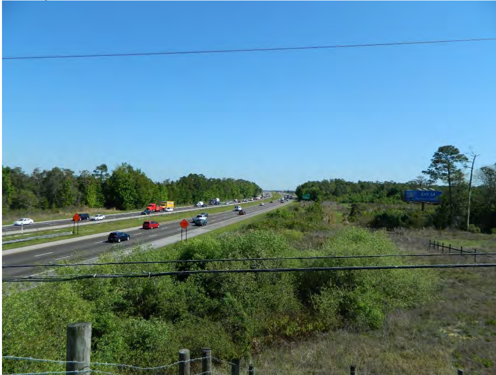
Looking NE along EB I-4 from Polk CR 54/Ronald Reagan Parkway overpass
