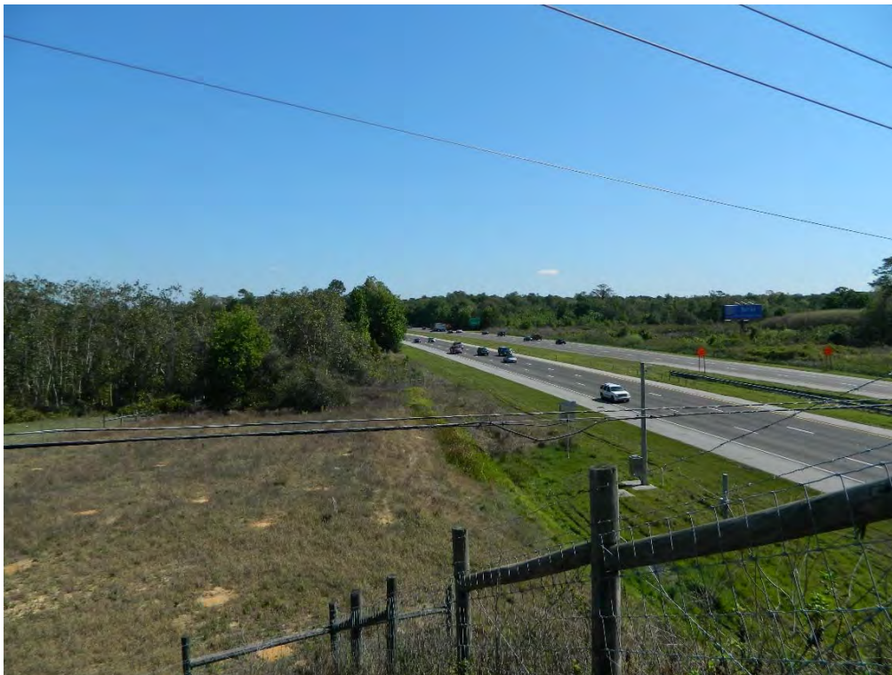
Looking NE along WB I-4 from Polk CR 54/Ronald Reagan Parkway overpass
