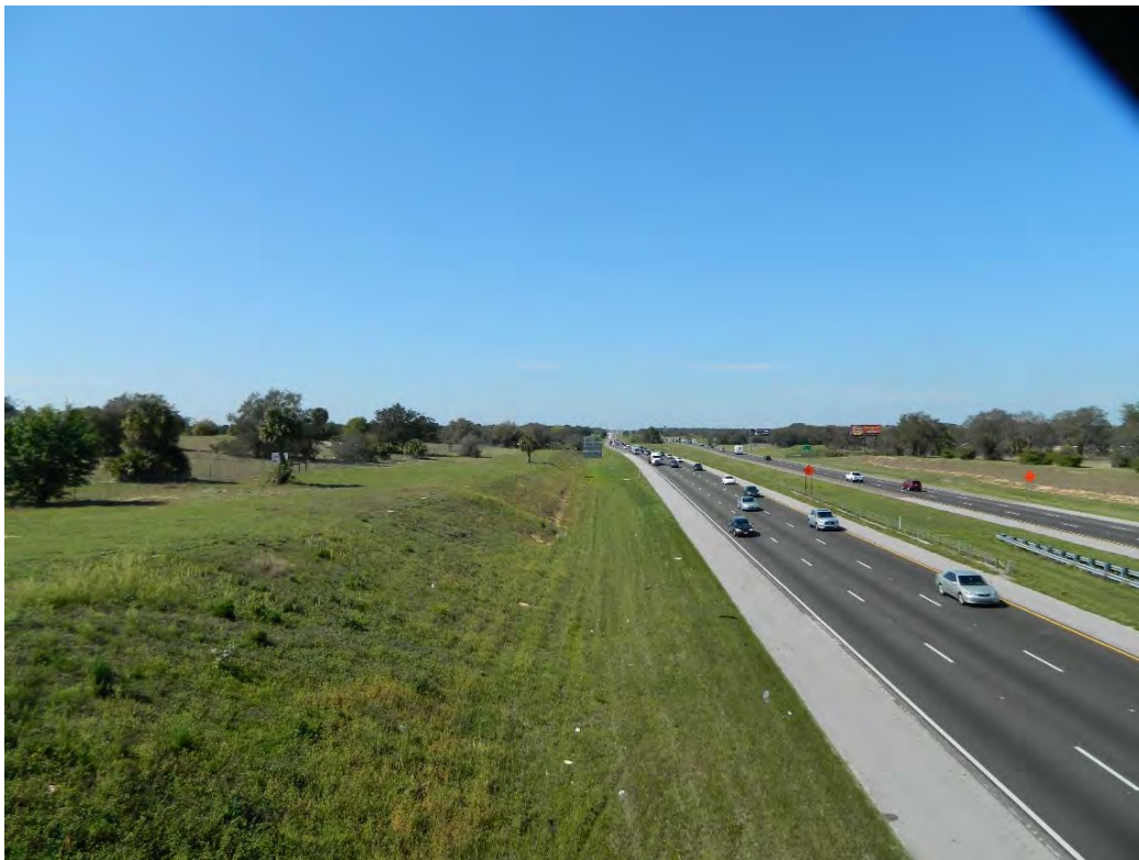
Looking SW along EB I-4 from Polk CR 54/Ronald Reagan Parkway overpass
