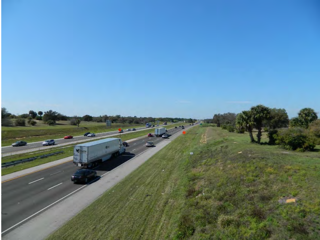
Looking SW. along WB I-4 from Polk CR 54/Ronald Reagan Parkway overpass
