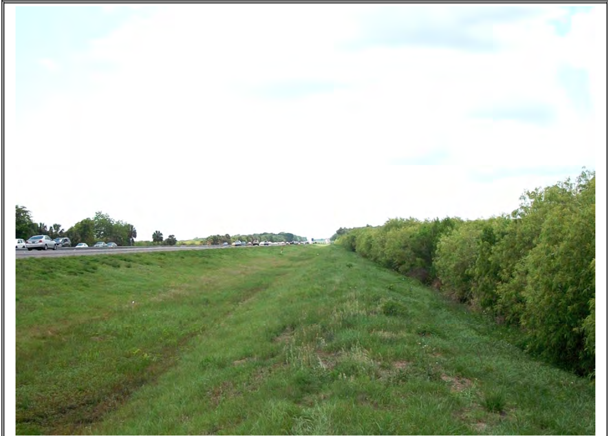
Treatment Swale 401-A Westbound
