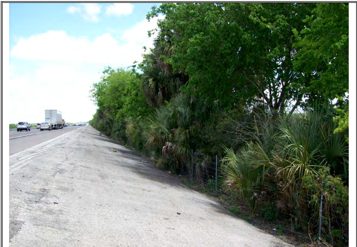
Treatment Swales 401-A Eastbound and 401-B
