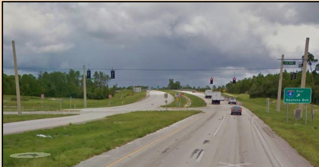
SR 472 Existing Street View
