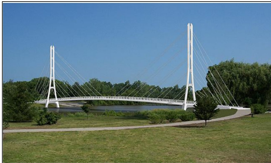
Figure 2: Representative Cable-Stayed Multi-Use Bridge
