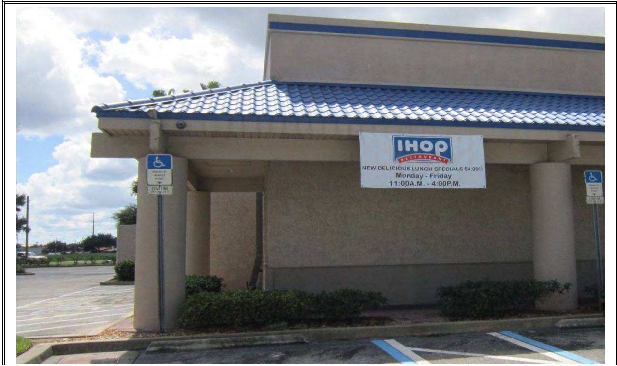
Site 218: IHOP Restaurant, formerly Mobil #02-DHW
