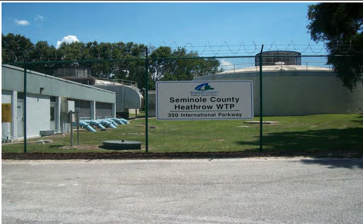
Site 146: Seminole County Heathrow WTP
