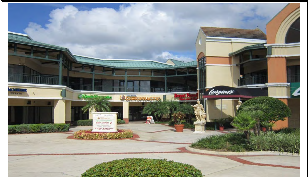
Site 134: Multiple Doctors' Offices B
