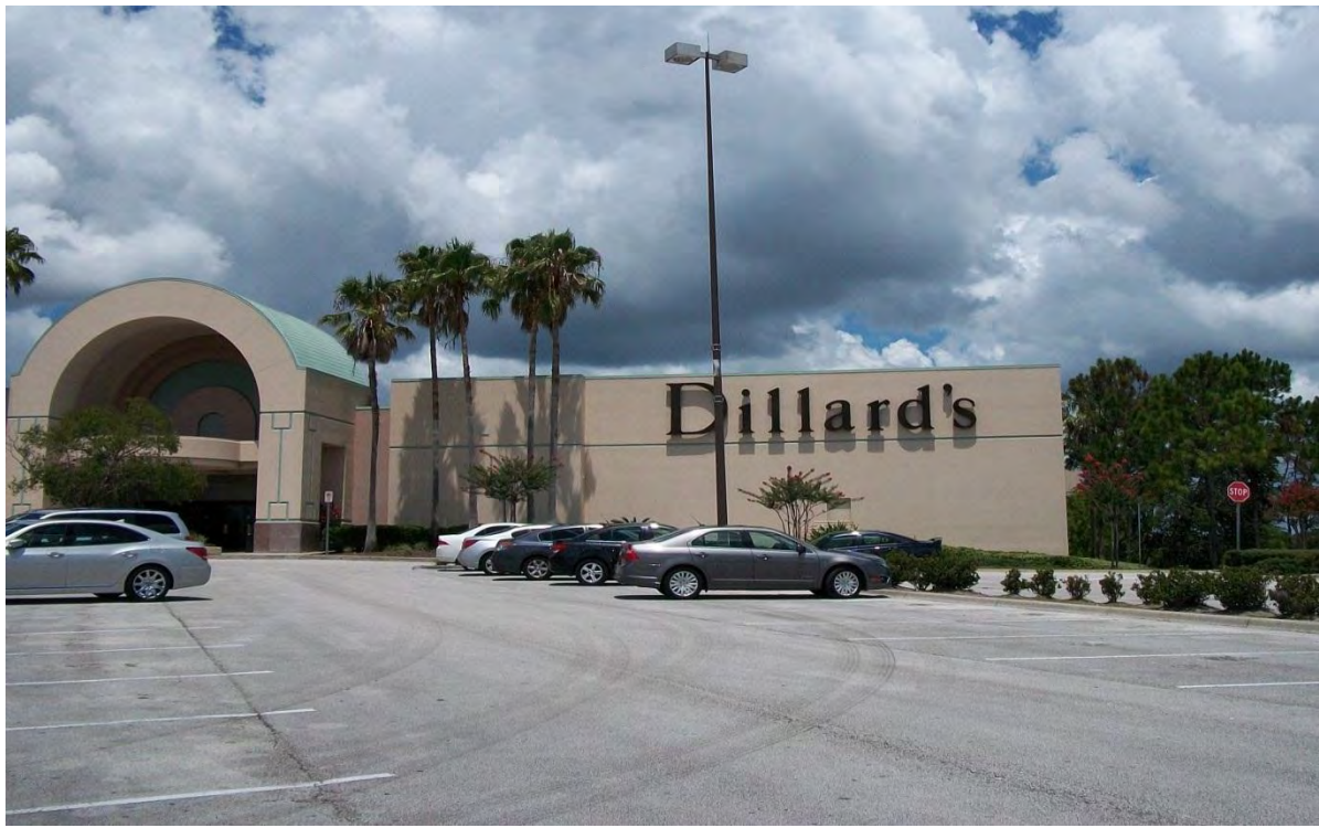
Site 210: Dillard's Department Store
