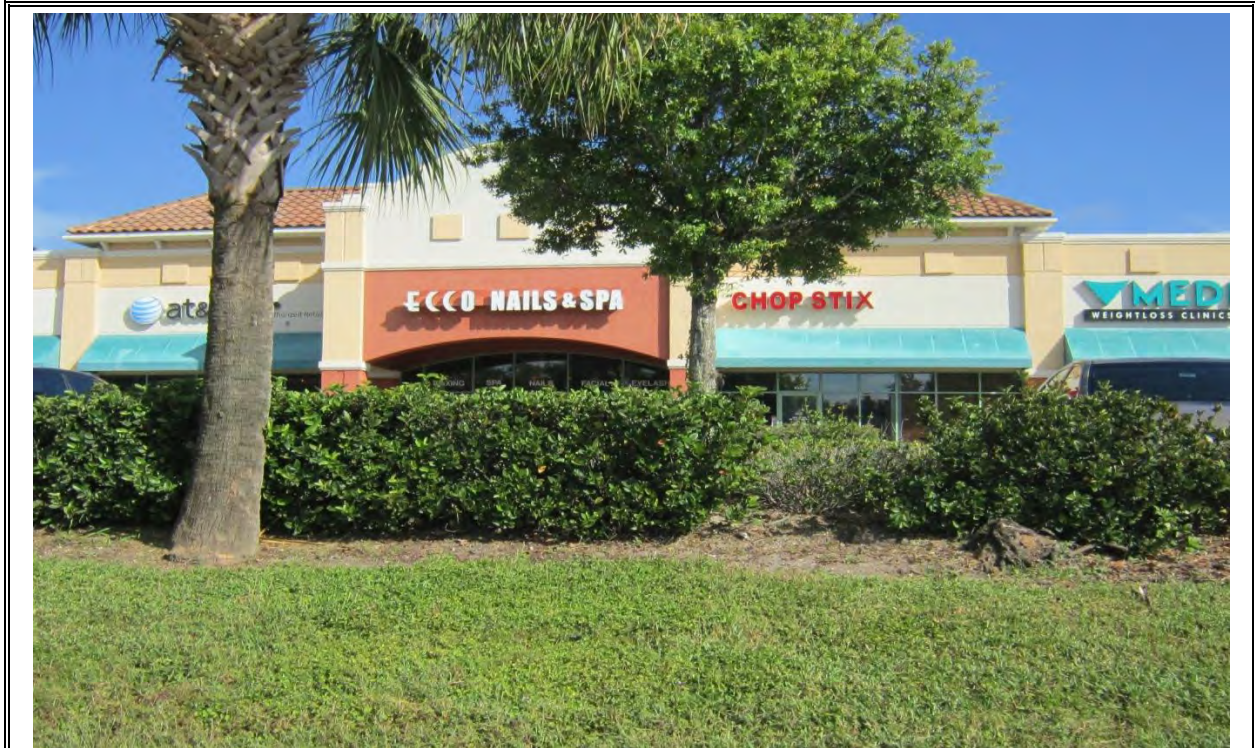
Site 132: Ecco Nails & Spa
