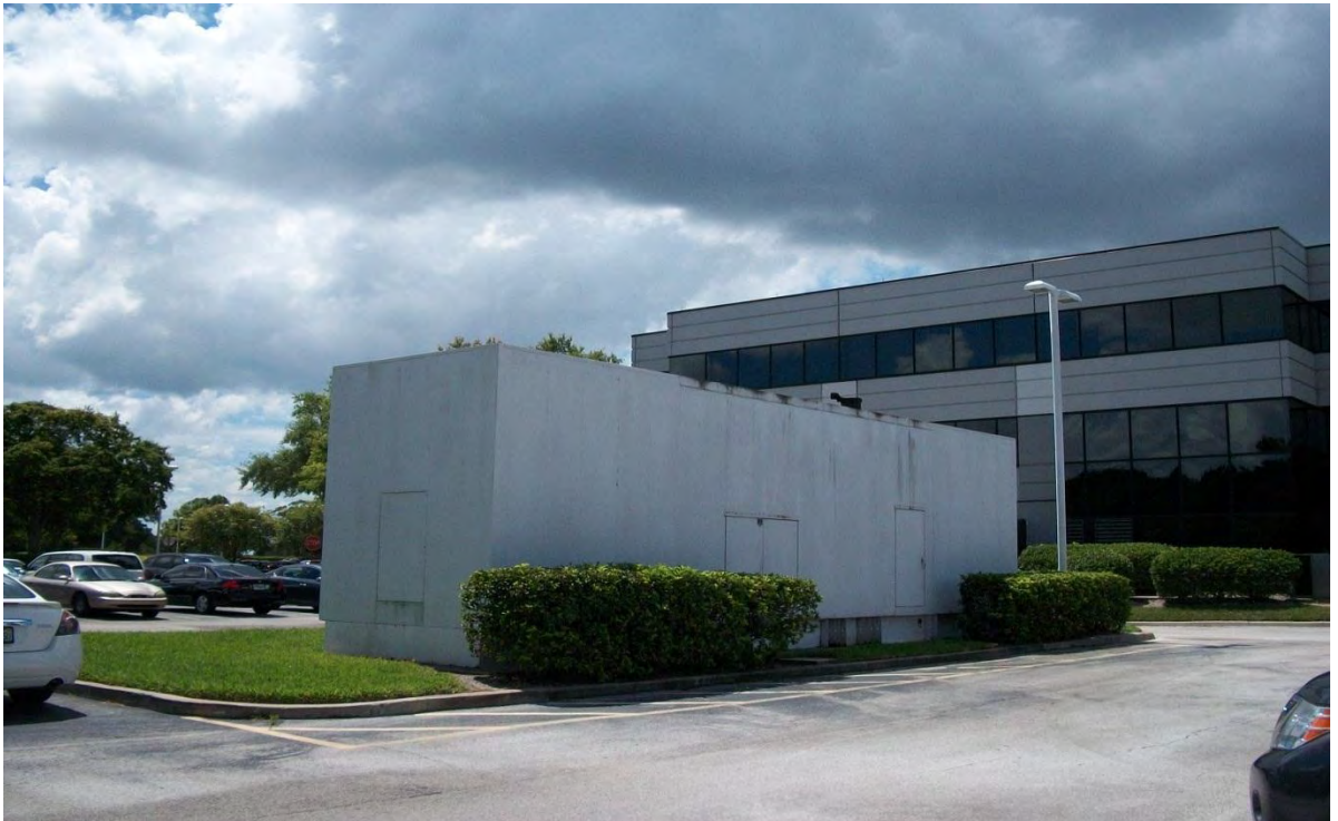
Site 93: Lake Emma Corporate Office Park
