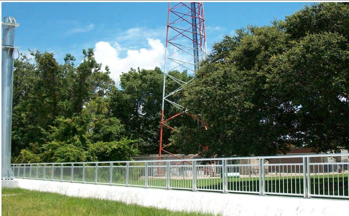
Site 217: Cell Tower with Diesel Generator E
