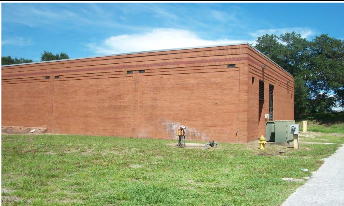
Site 150: Bellsouth Telephone Inc. #39280
