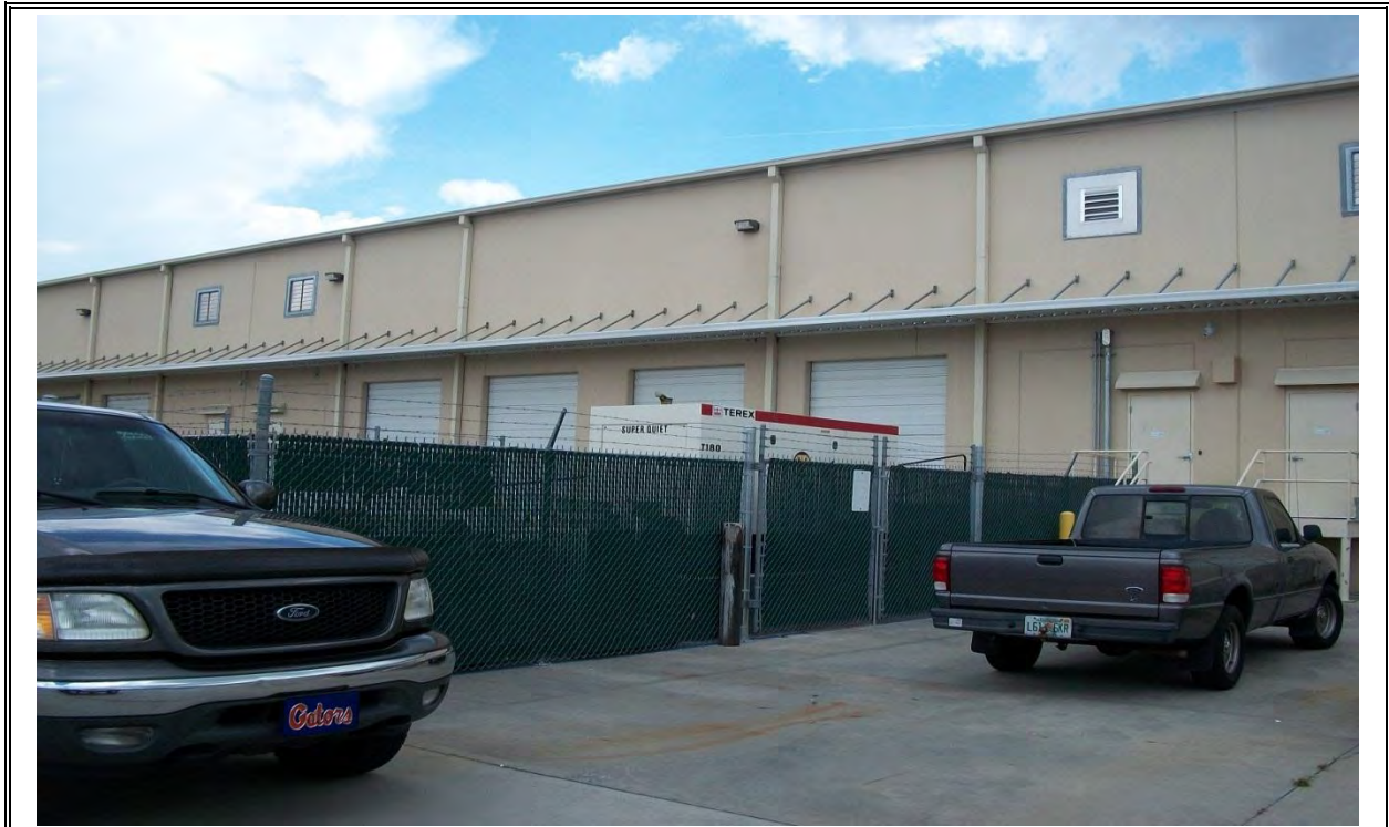
Site 269: Omnicare of Central Florida
