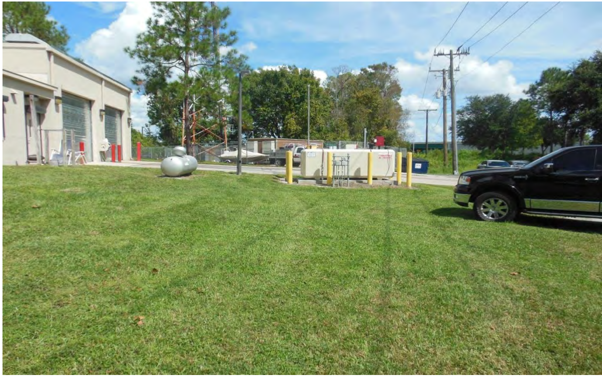
Site 216: Seminole County Fire Station #34
