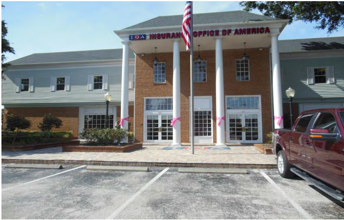
Site 27: Former Site of R & R Truck Sales INC
