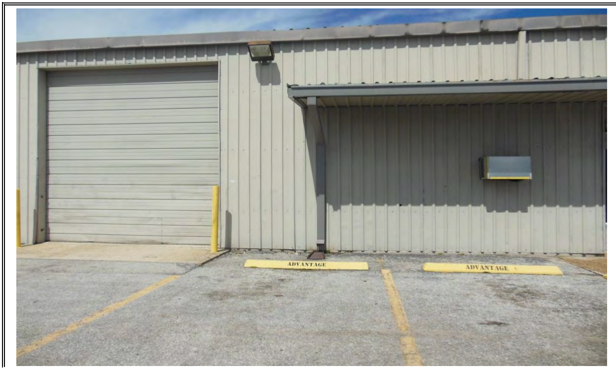
Site 243: Former Site of Macedo Motorsports
