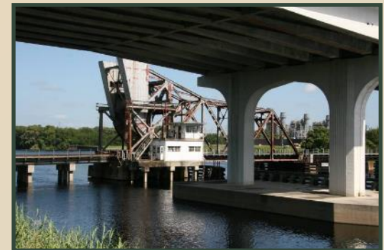
Resource 8SE02823, ACL Railroad Bridge over St. Johns River.
