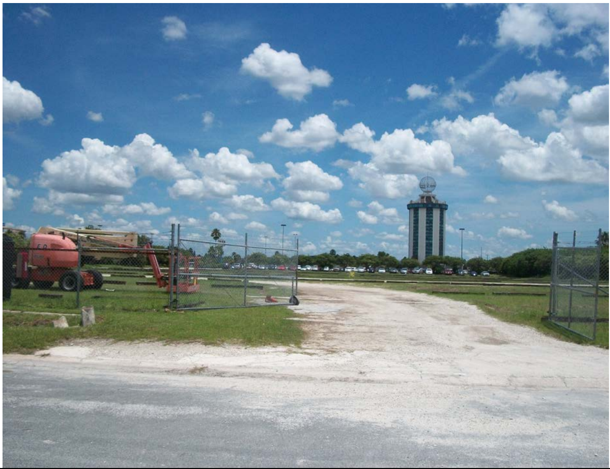
Site 96: Wet 'n Wild, former site of Power Concrete Products Company
