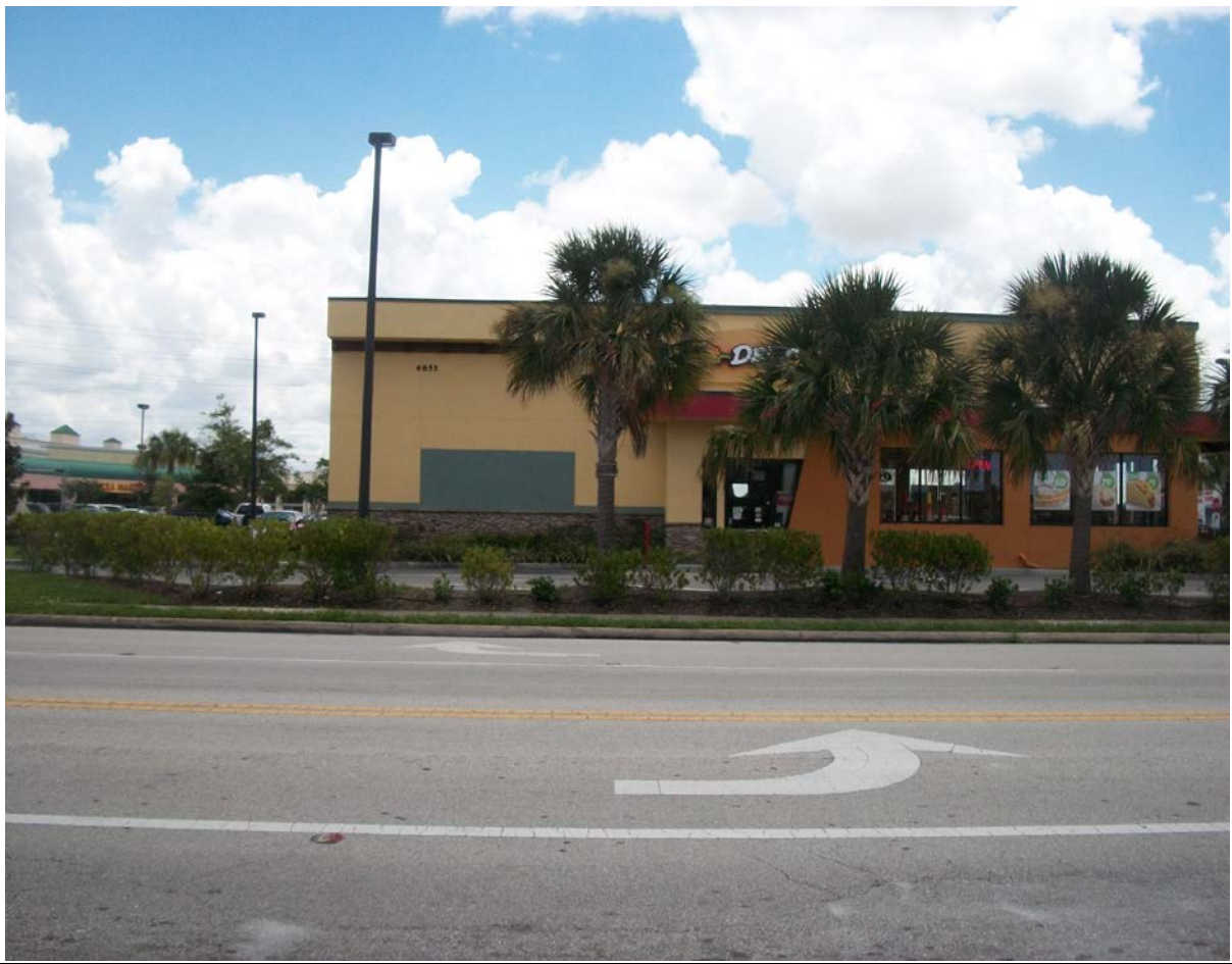
Site 108: Del Taco, Formerly Exxon #40262
