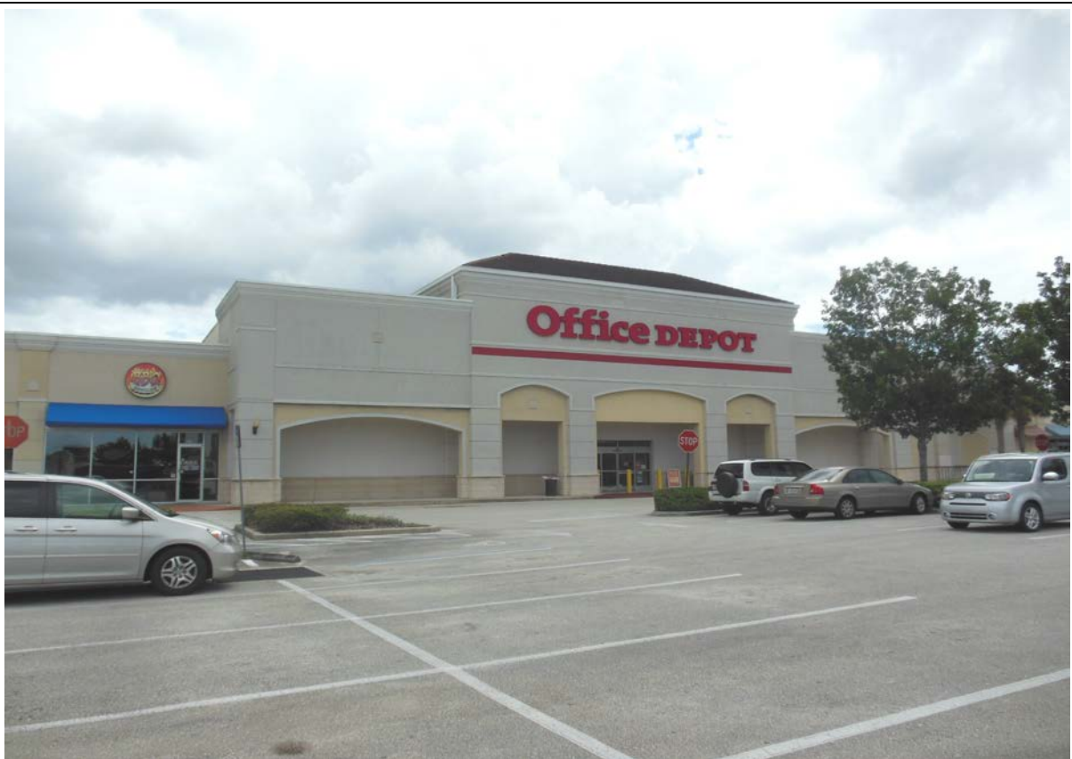
Site 107: Office Depot #553
