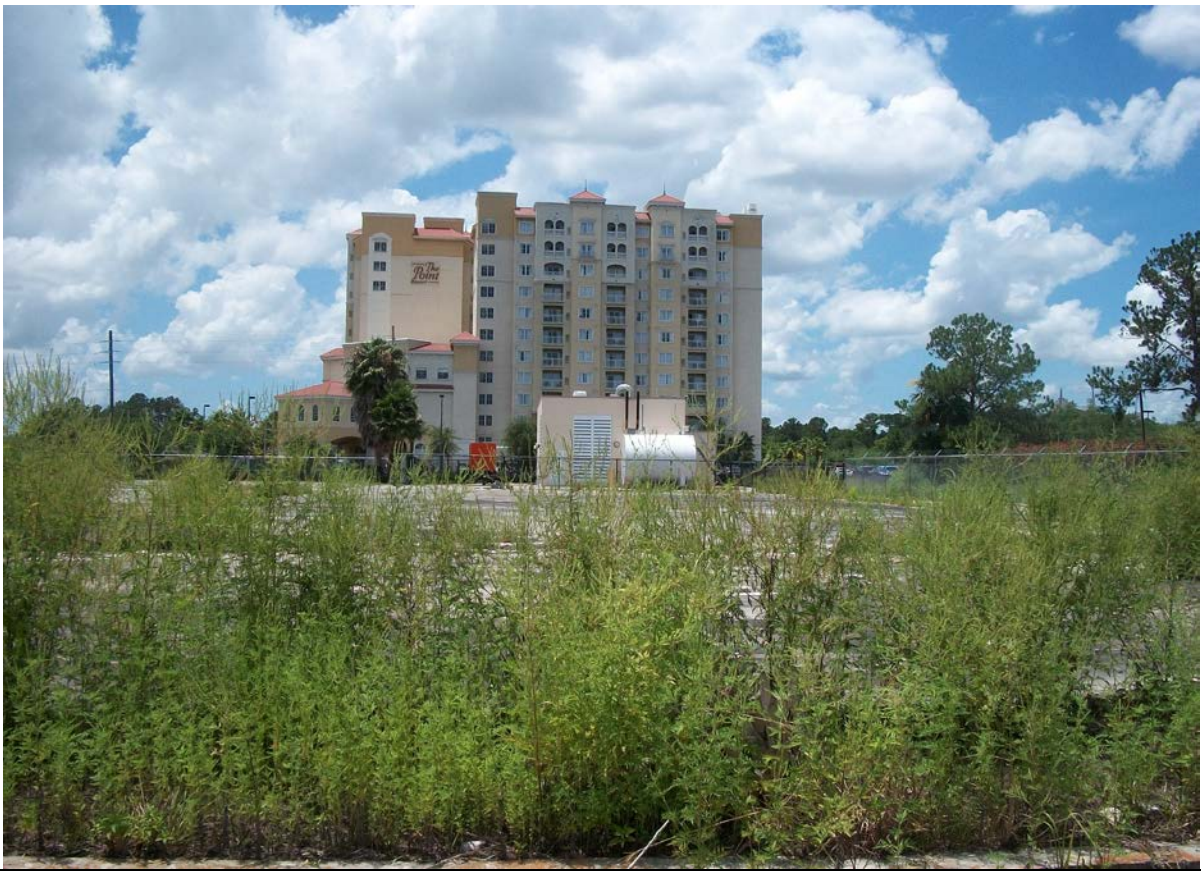
Site 94: Orlando City Lift Station #29
