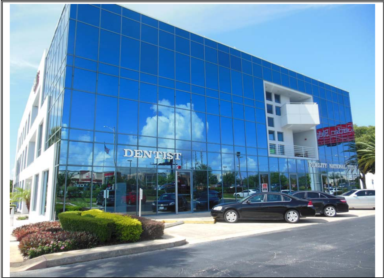
Site 64: Multiple Doctors' Offices D
