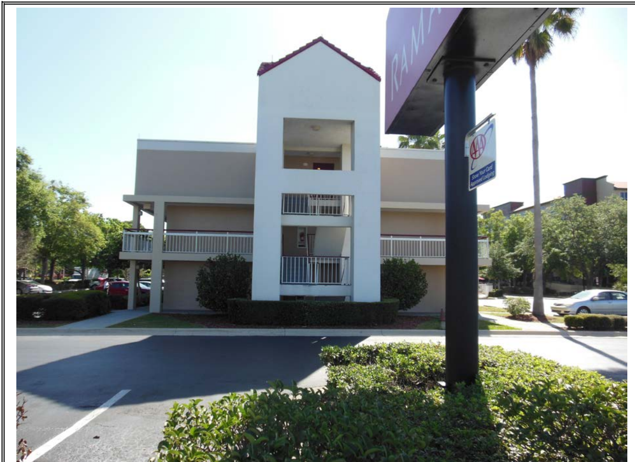
Site 53: Ramada Inn
