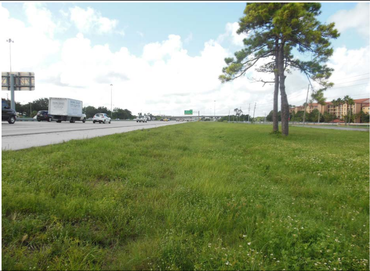
Site 22: GT Specialists Spill Site – Looking westbound toward the I-4/SR-528 Interchange
