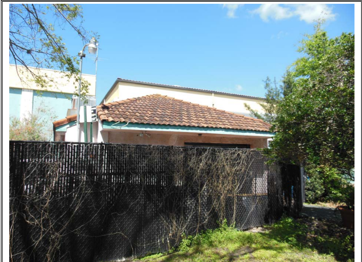
Site 51: YMCA – Pool chemical storage
