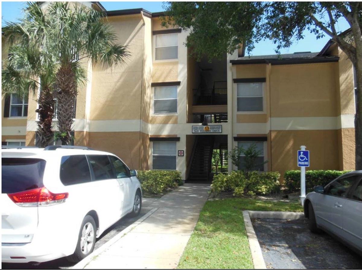
Site 44: Former Debernardi Printing
