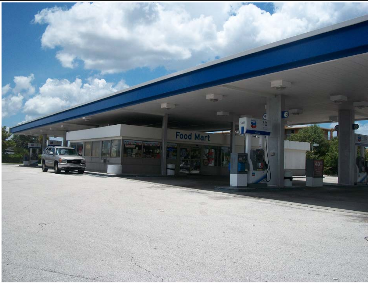
Site 104: Chevron International, former Shell
