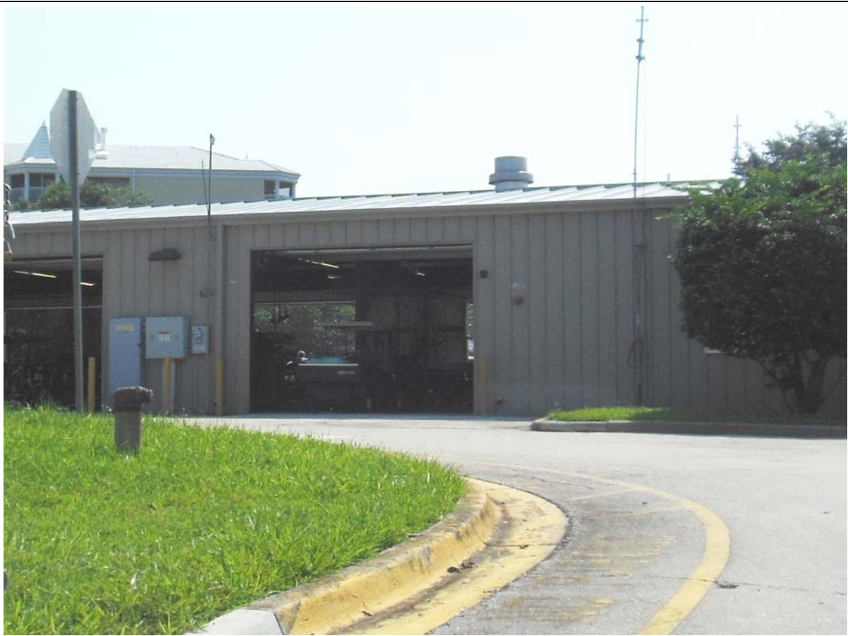
Site 1: Marriott Cypress Pines Golf Course Maintenance Facility
