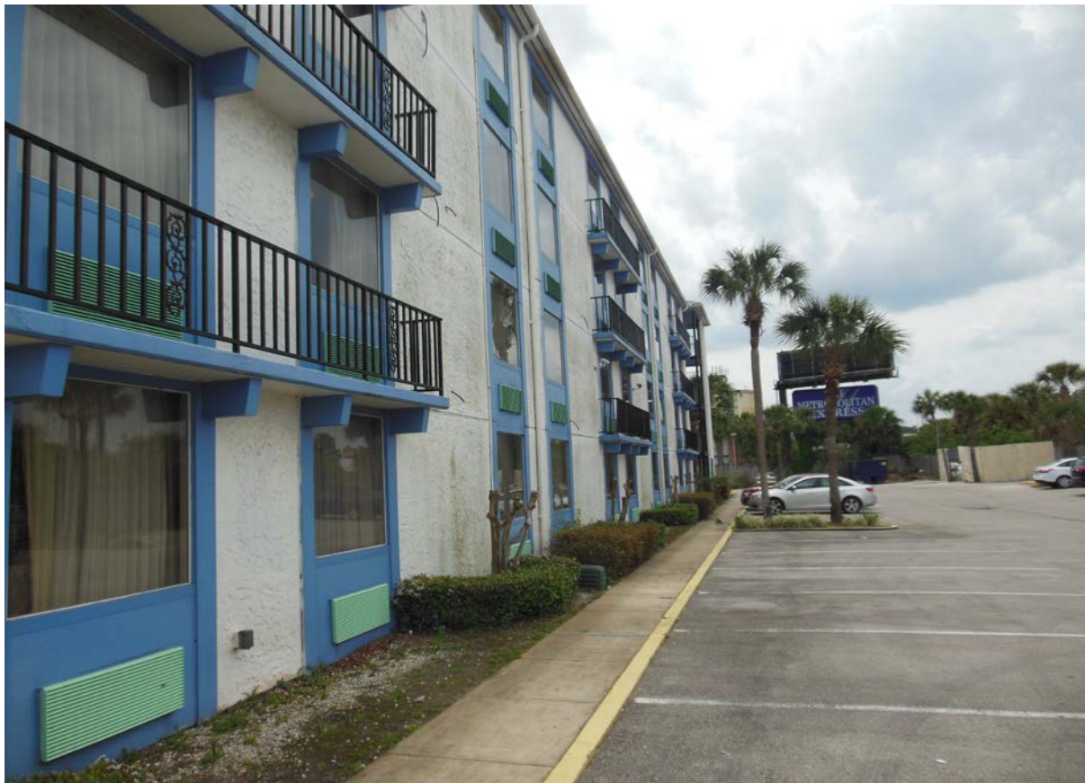
Site 102: Orlando Monumental Movieland Hotel – north side of building, facing west, dumpster and chemicals at right side of picture
