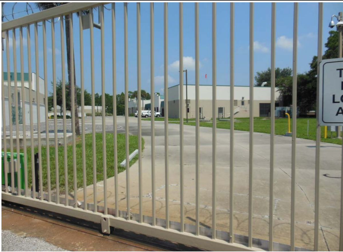
Site 110: Orlando Utility Commission SW Water Plant
