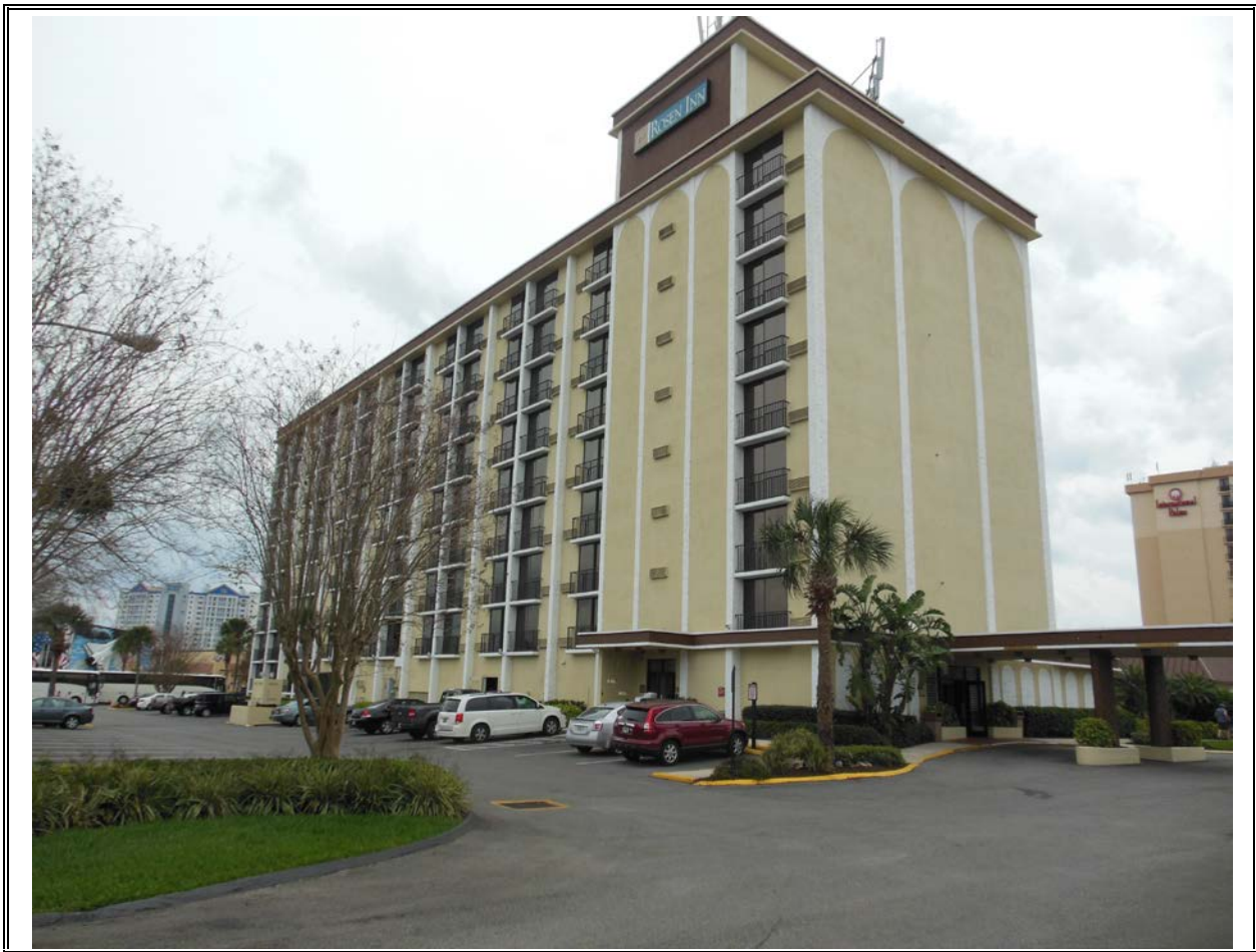
Site 99: Rosen Inn – northwest corner of building, facing southeast
