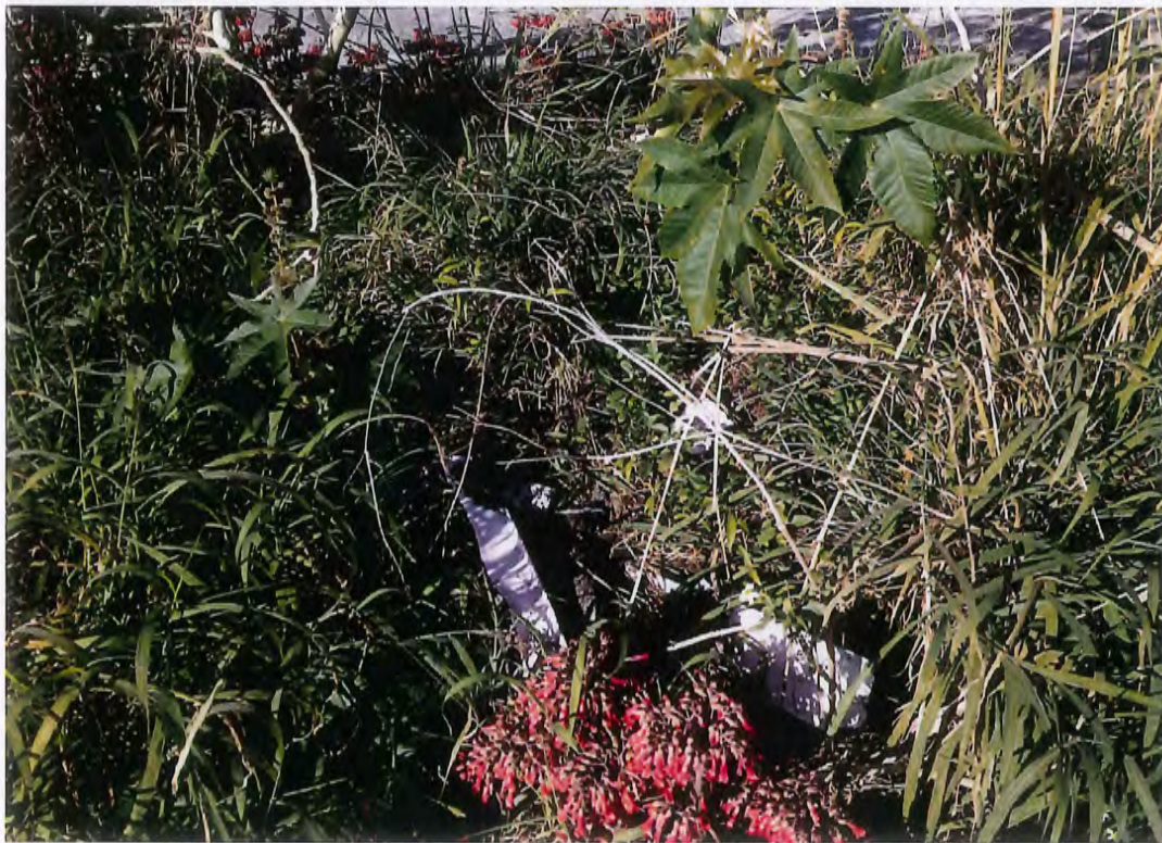
2. View of metal drip edge and shingles located in Debris Pile #1.
