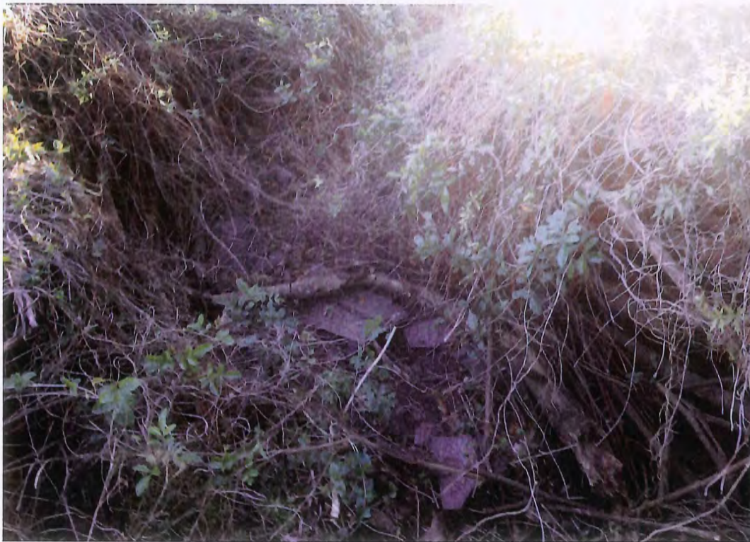
16. View of homogeneous area BDP1-1, gray asphalt shingles, located beneath the vegetation in Building Debris Pile #1. No asbestos was detected in homogeneous area BDP1-1.
