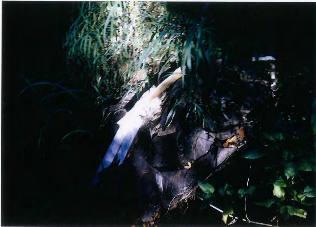
7. View of homogeneous area DP2-2, brown asphalt shingles, located in Debris Pile #2. No asbestos was detected in homogeneous area DP2-2.
