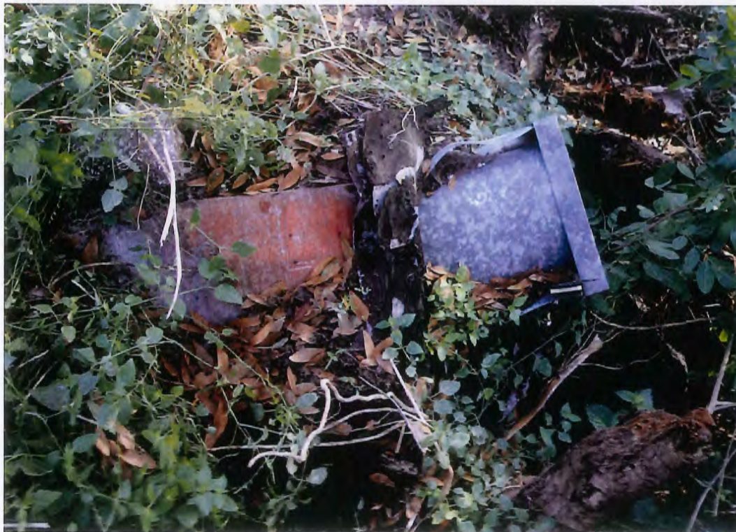
6. View of homogeneous area DP2-1, chimney flashing, located in Debris Pile #2. Laboratory analytical results showed 5% chrysotile asbestos in homogeneous area DP2-1.
