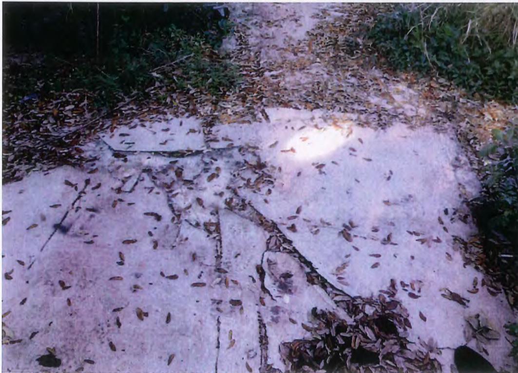
22. View of homogeneous area SLAB, vinyl sheet flooring (VSF) with rock pattern located on the slab. Analytical results showed 20% chrysotile asbestos in homogeneous area SLAB.
