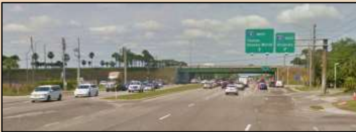
SR 482 Existing Street View
