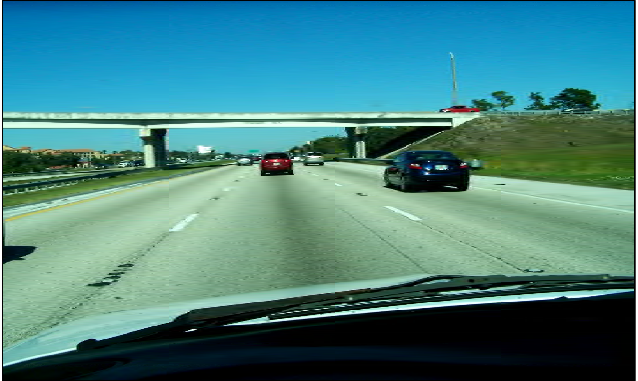
Photo 1: I-4 eastbound near MP 6.305. Typical condition of the mainline lanes between MP 6.018 to MP 6.482.
