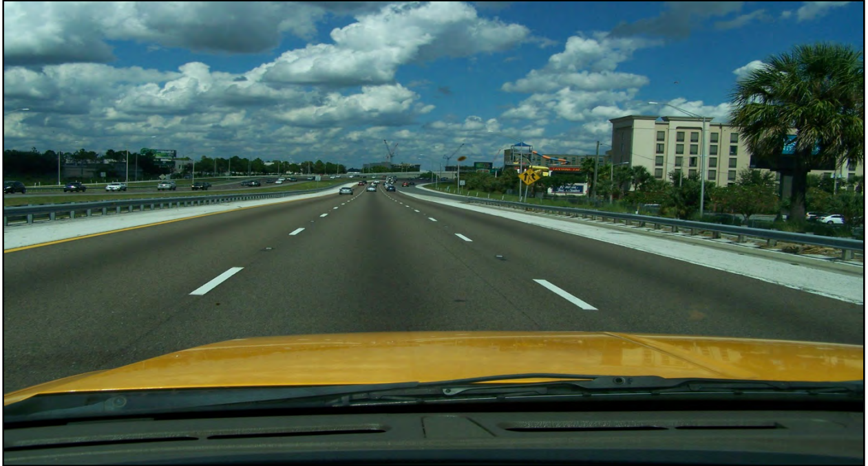
Photo 9: I-4 eastbound near MP 8.400. This location between MP 8.264 and MP 8.844 was resurfaced in 2007. Note the granite open-graded friction course.
