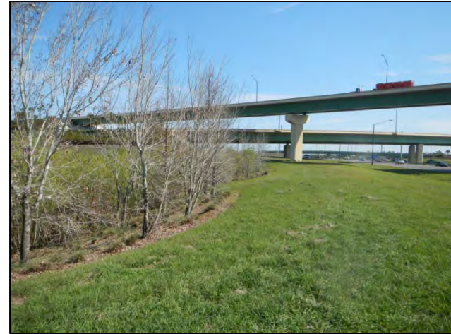
Area 21 facing NE
