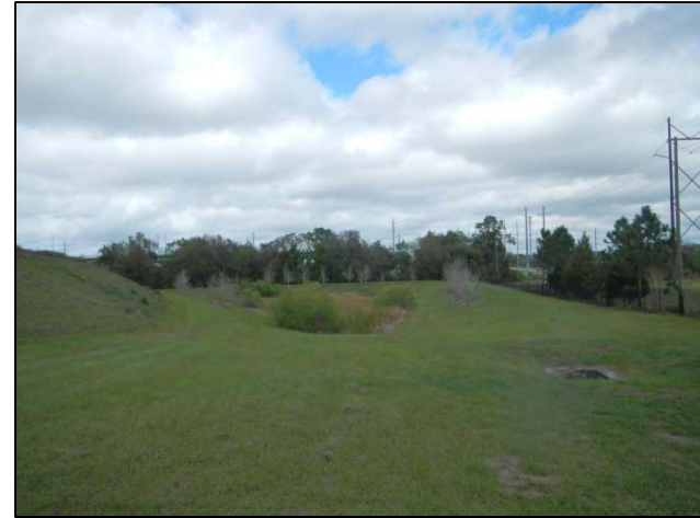
Area 8 facing NE
