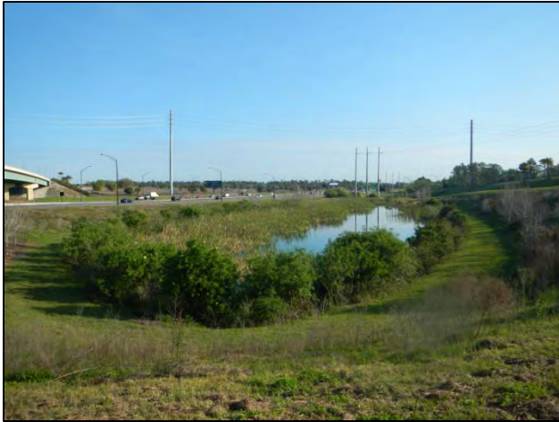
Area 11 facing NE
