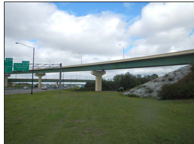
Area 9 facing NE
