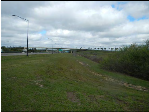
Area 9 facing NE
