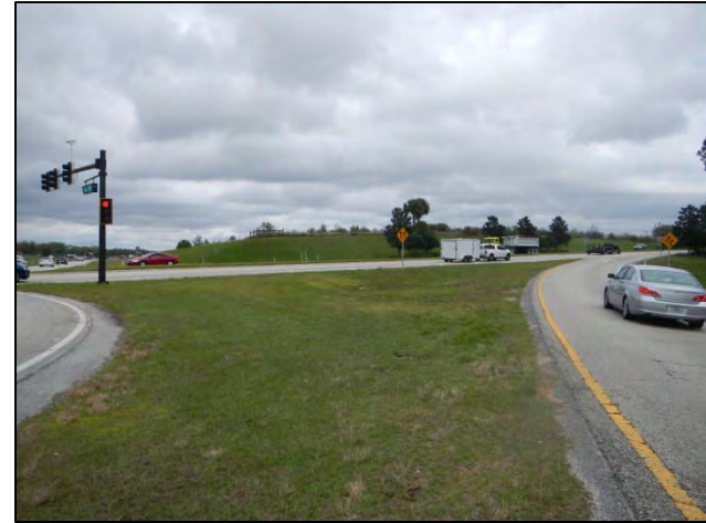
Area 2 facing NE
