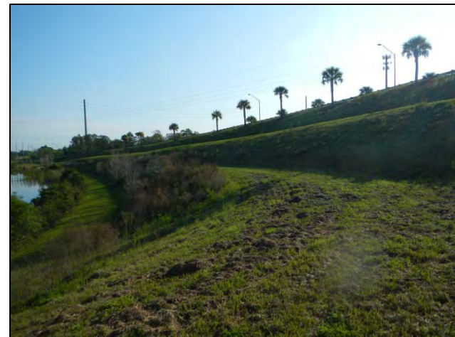
Area 11 facing E
