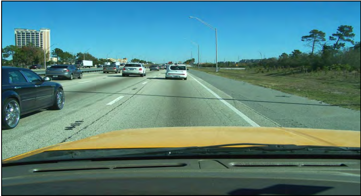
Photo 2: I-4 eastbound near MP 2.359. Note the fair condition of the outside paved shoulder and a continuous longitudinal crack at a construction joint between the R2 and R3 lanes.
