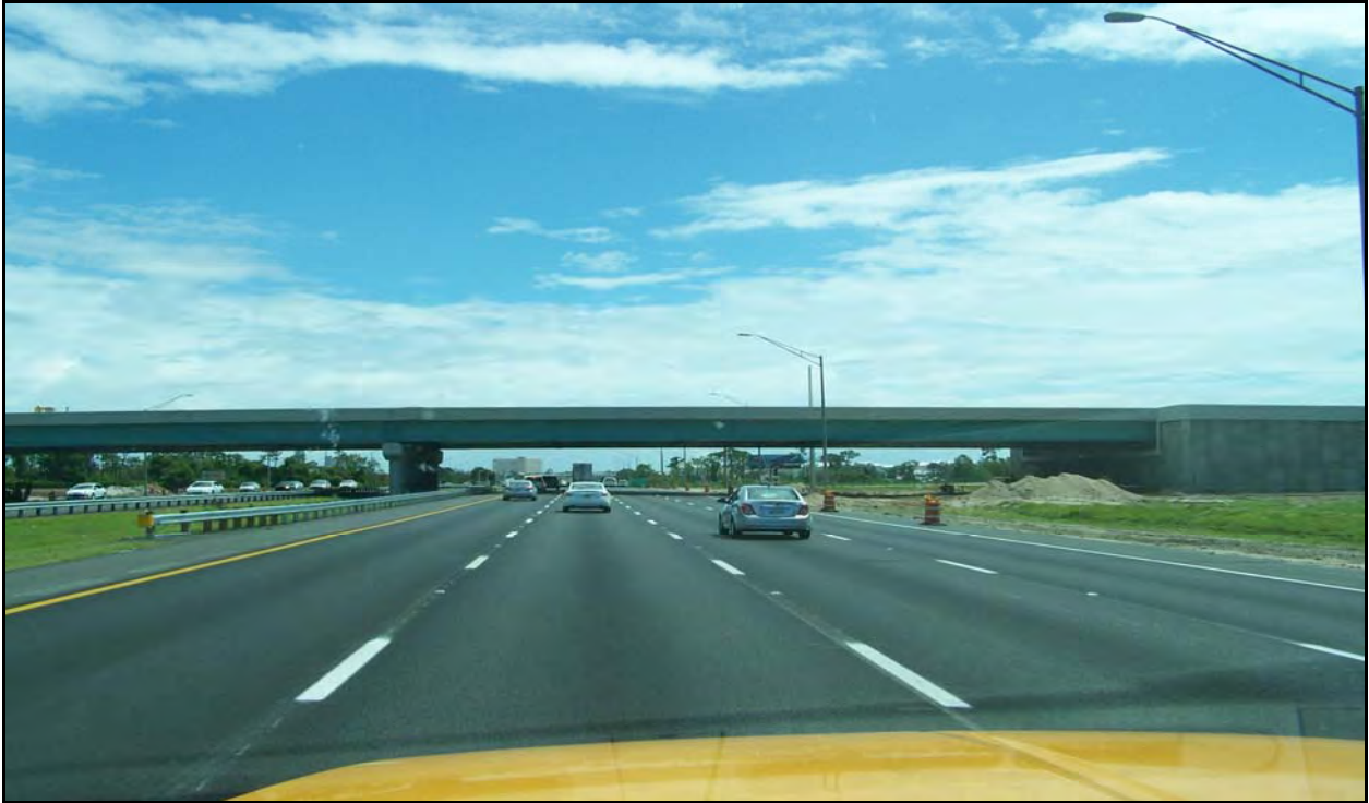
Photo 4: I-4 eastbound near MP 4.300. This photo shows the pavement condition from MP 4.074 to MP 4.607 that will not be an exception to rehabilitation. The mainline lanes were only milled 0.75 inches and resurfaced with FC-5 only.
