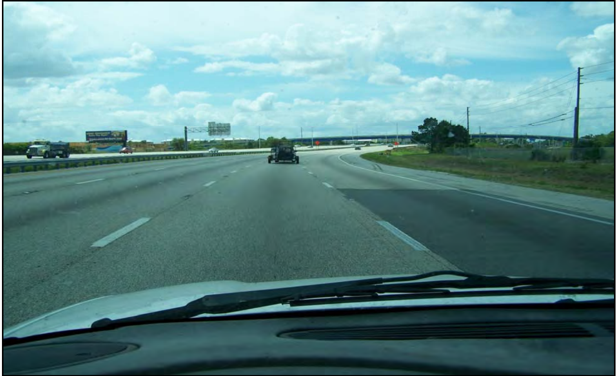
Photo 9: I-4 westbound near MP 5.788. Typical condition of the westbound roadway.
