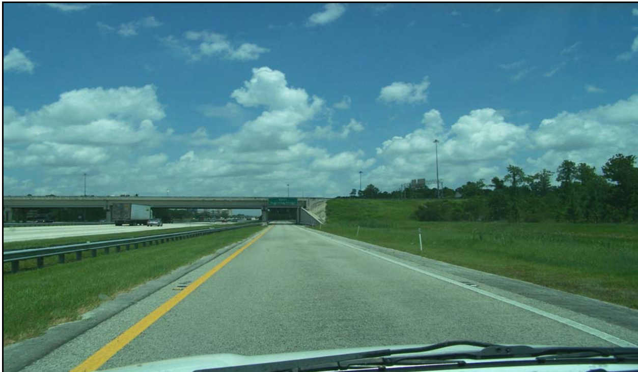
Photo 6: I-4 westbound on Ramp 75039-008. This is the ramp from I-4 eastbound to SR 536 westbound.
