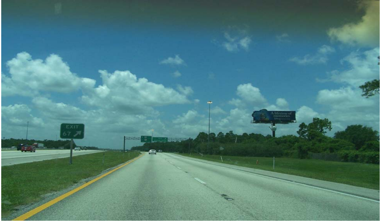
Photo 5: I-4 westbound on Ramp 75280-127. This photo shows the relatively fair condition of this connector ramp. Note that the outside shoulder is not paved with an open-graded friction course.
