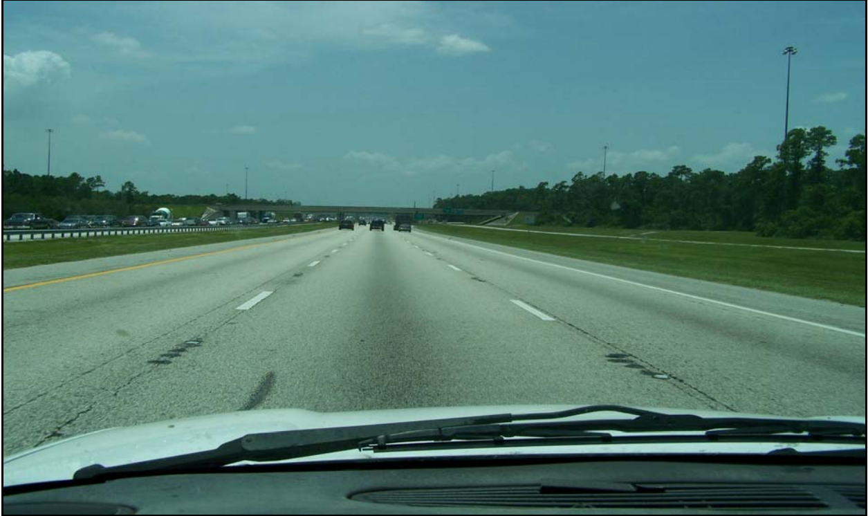
Photo 4: I-4 westbound near MP 1.423. The westbound lanes are not in as degraded condition as the eastbound lanes. The mainline lanes of I-4 within the project limits are tangent with no curves. Our milling recommendations for the westbound lanes are for the long-term pavement preservation of the existing pavement.
