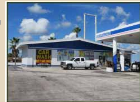
Resource 8PO07962, ca. 1967 Masonry Vernacular Building
