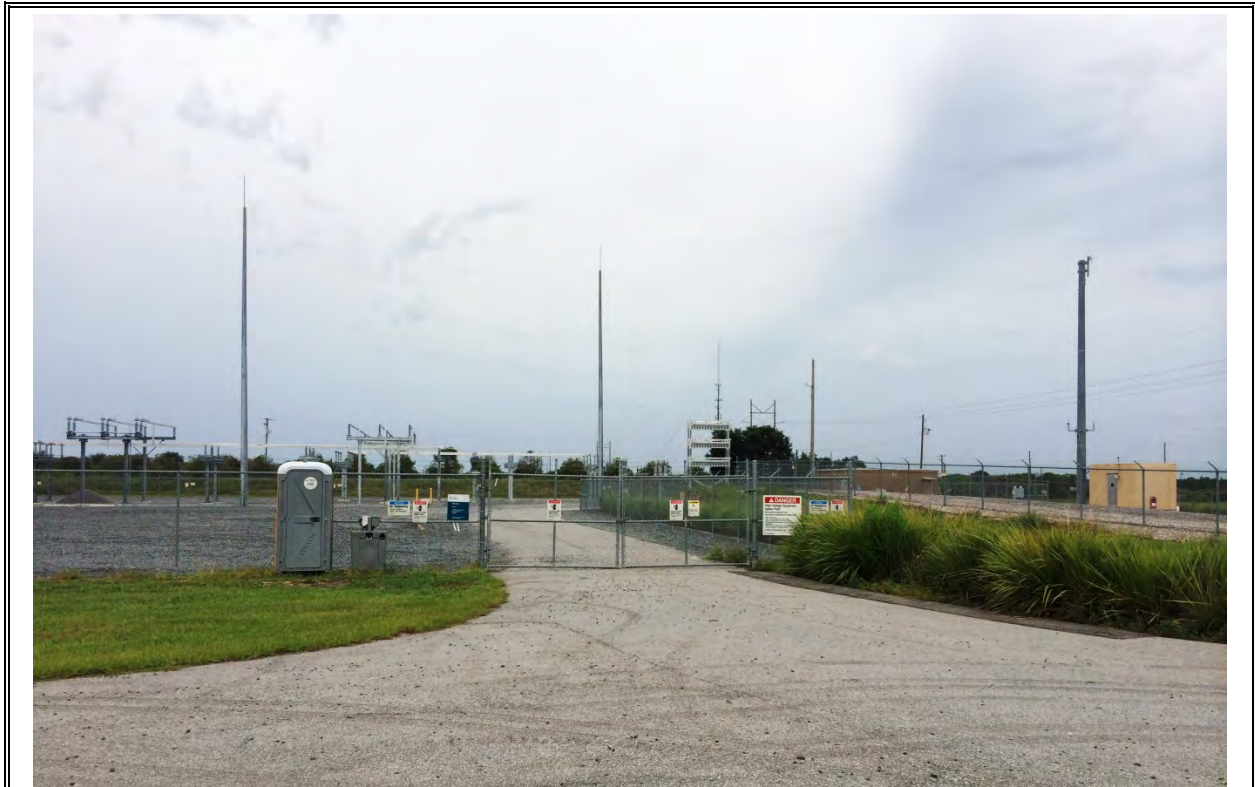
Site 3: Northridge Substation and Baseball City Meter Station
