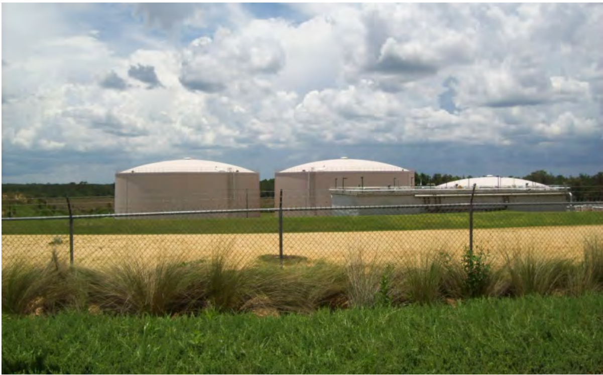
Site 5: Polk County Utilities Division NE Region WWTF
