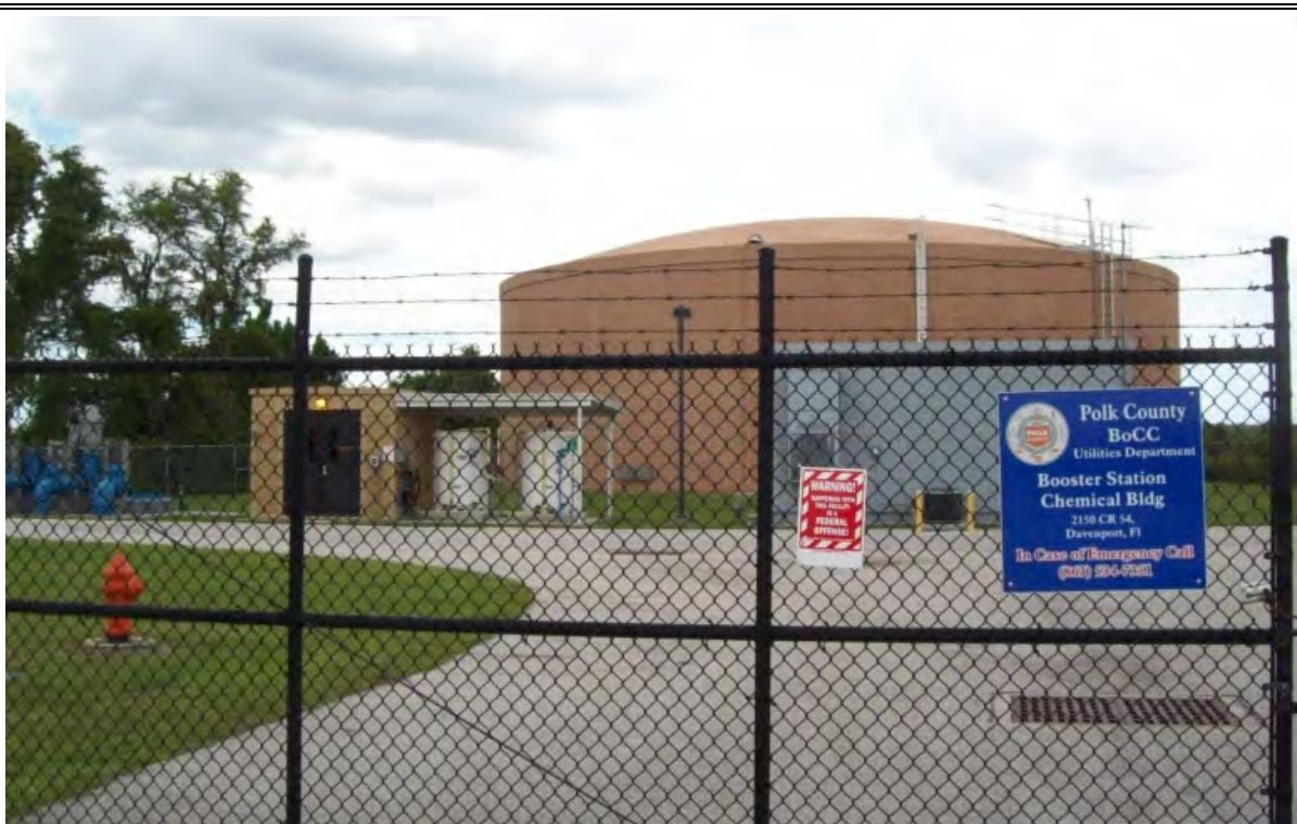
Site 38: Polk County Utilities Booster Station Chemical Building
