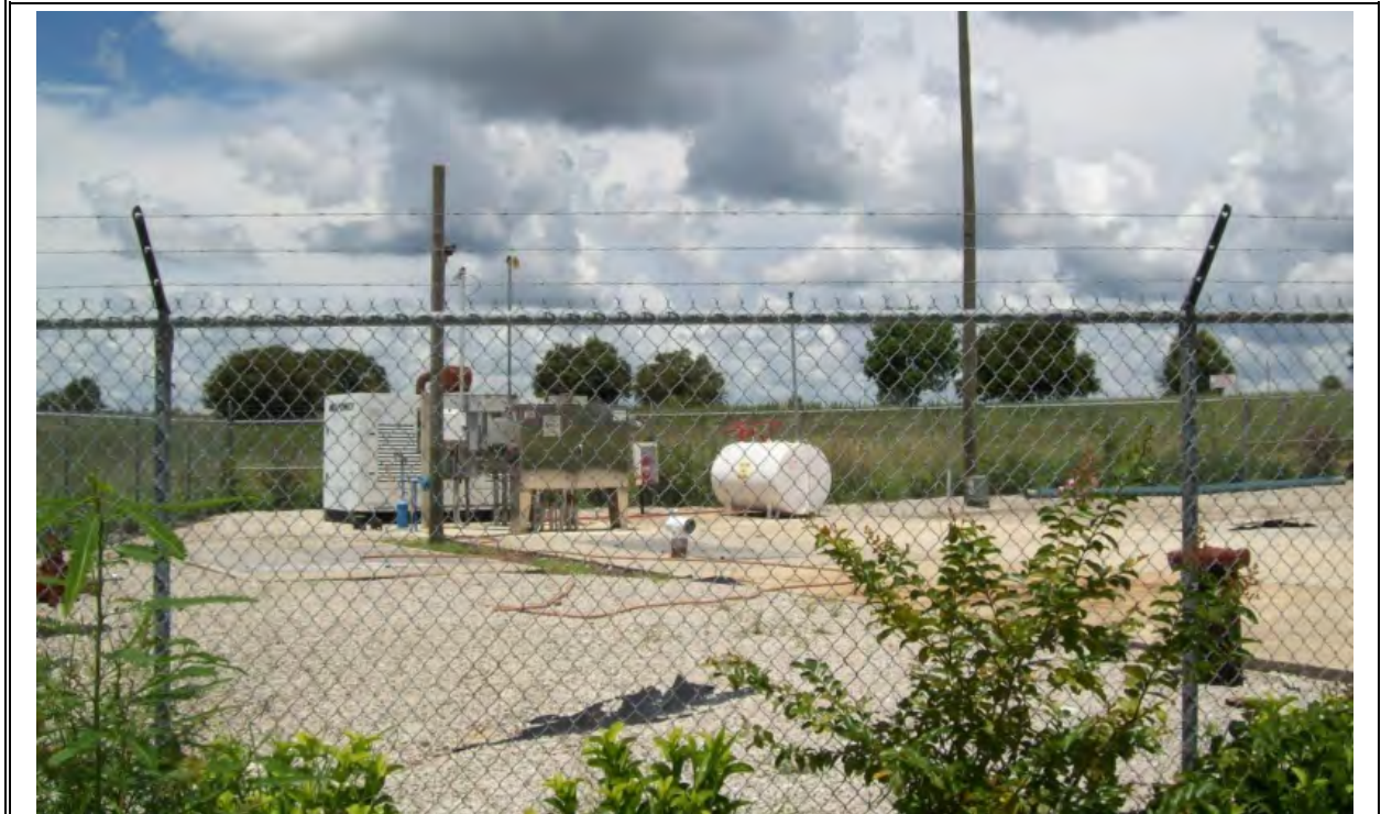
Site 31: Polk County Utilities NE Lift Station #106
