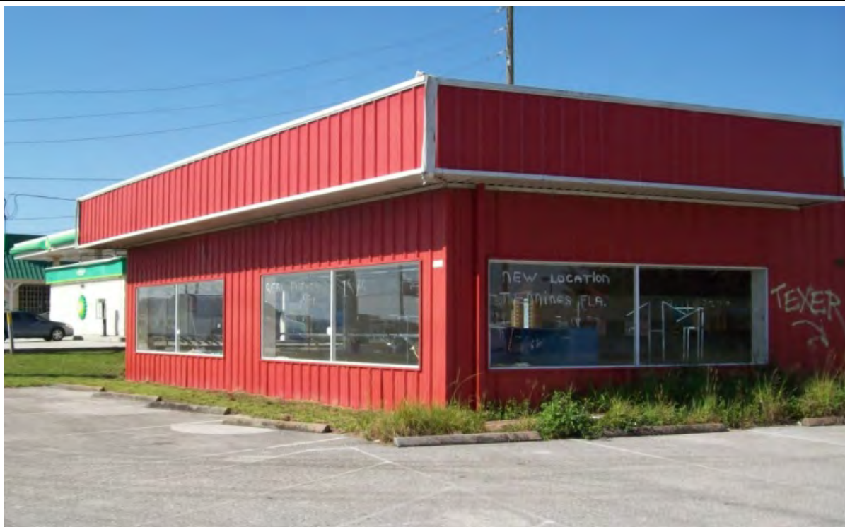
Site 15: Vacant Parcel, formerly Chevron #47333, John's Mini Mart
