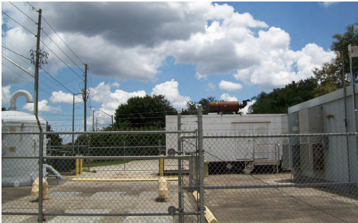
Site 37: Lift Station with Diesel Powered Emergency Generator
