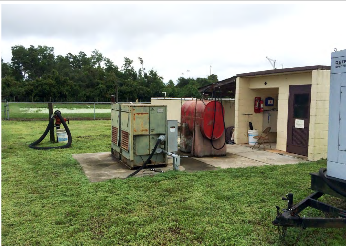
Site 98: Four Towns Wastewater Treatment Plant
