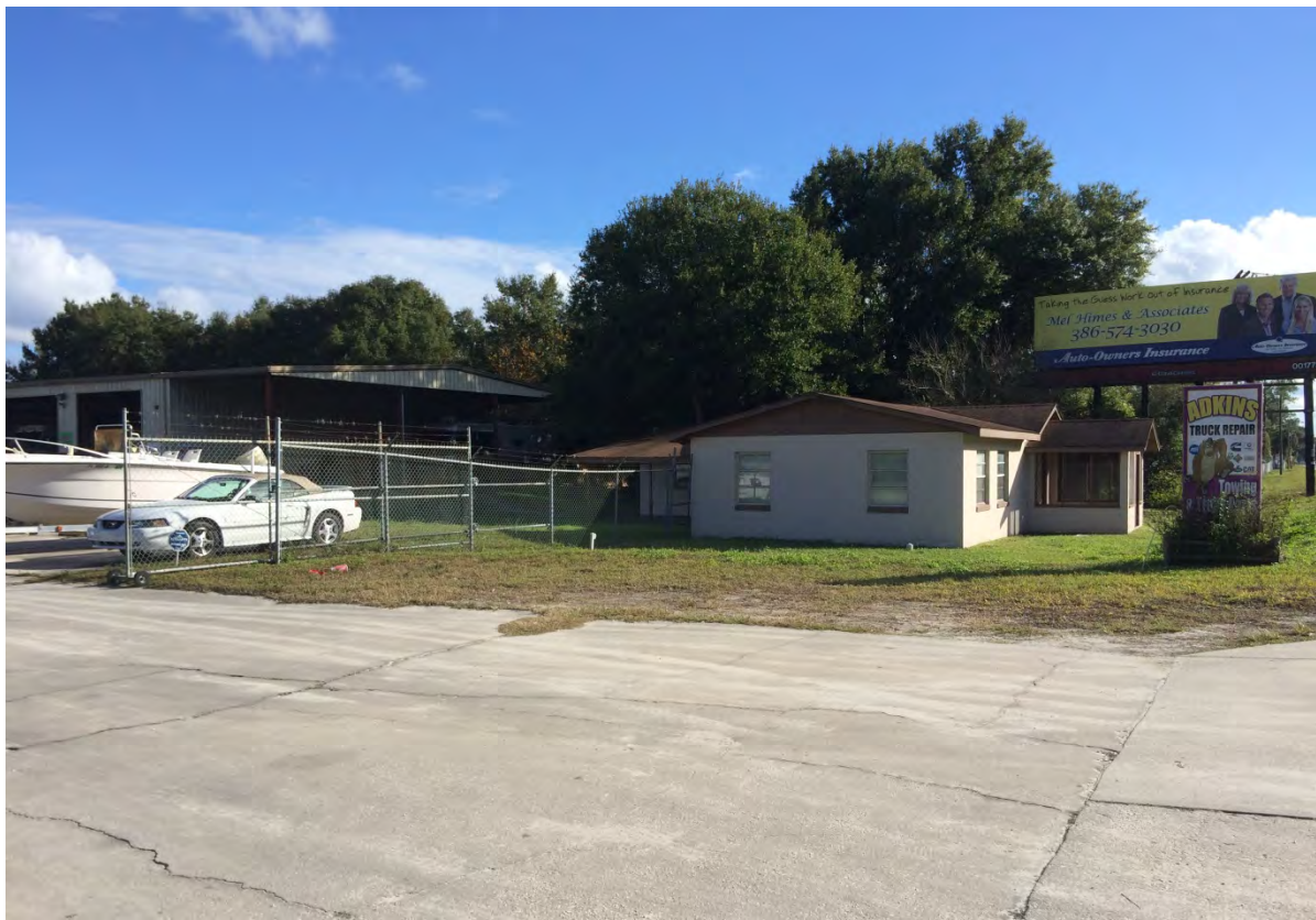
Site 7: Adkins Truck Repair, formerly Sunbelt Auto Carriers
