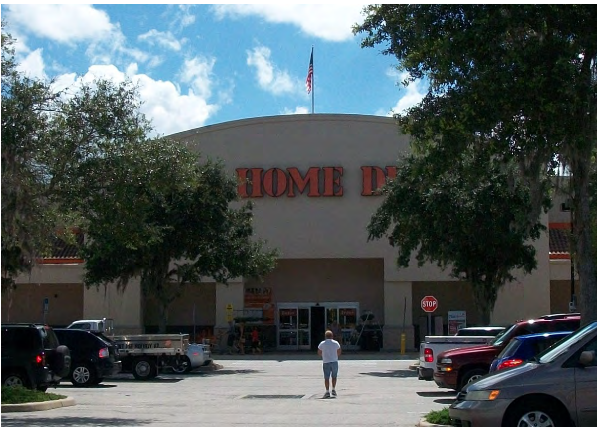
Site 86: Home Depot #6323
