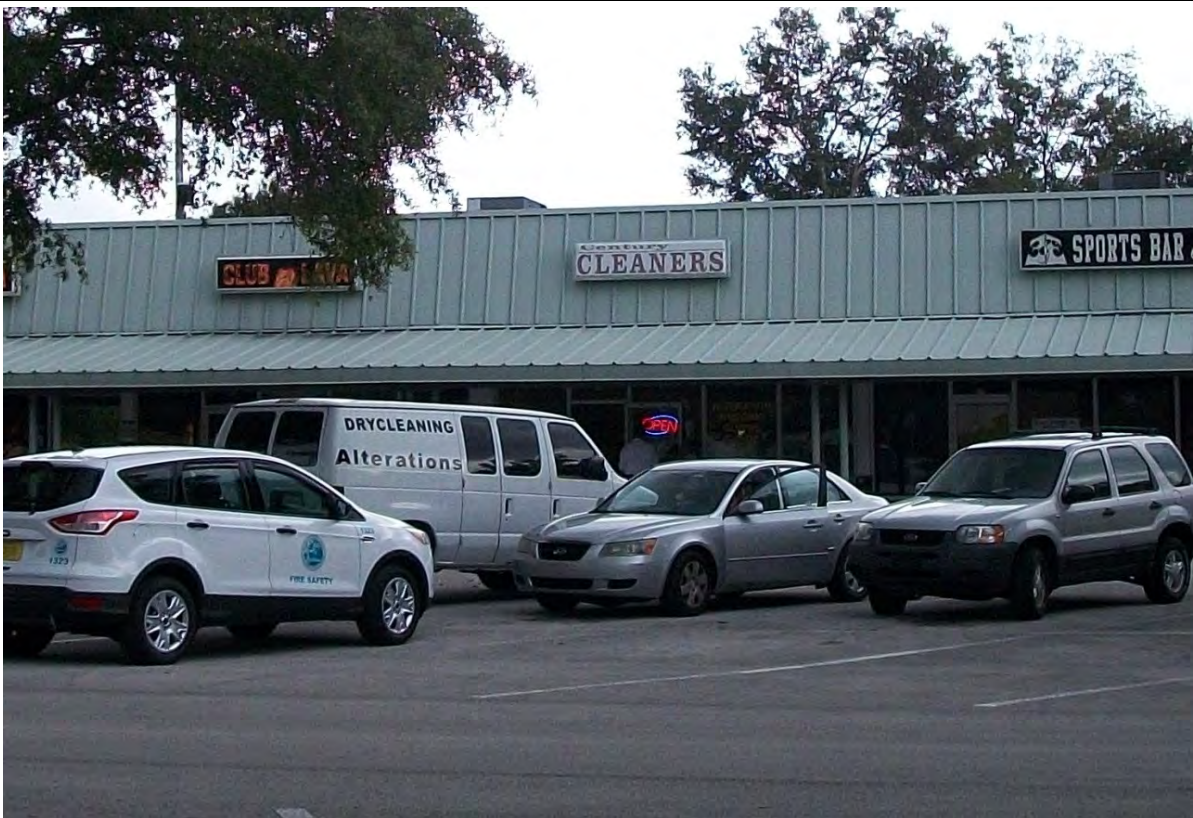
Site 54: Deltona Plaza Multiple Businesses
