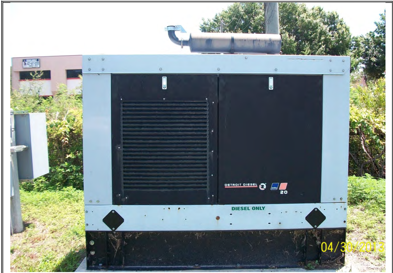
Site 15: FDOT Diesel Powered Generator
