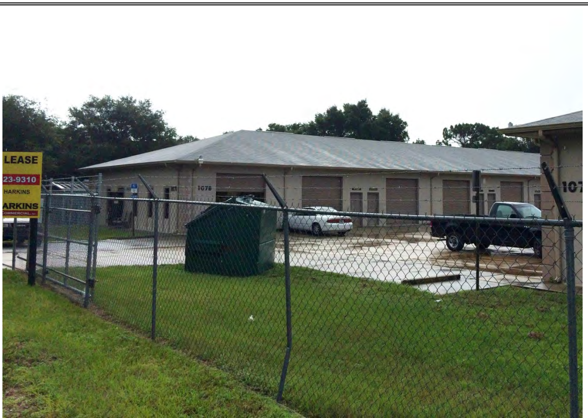
Site 120: Gator Radiator LLC
