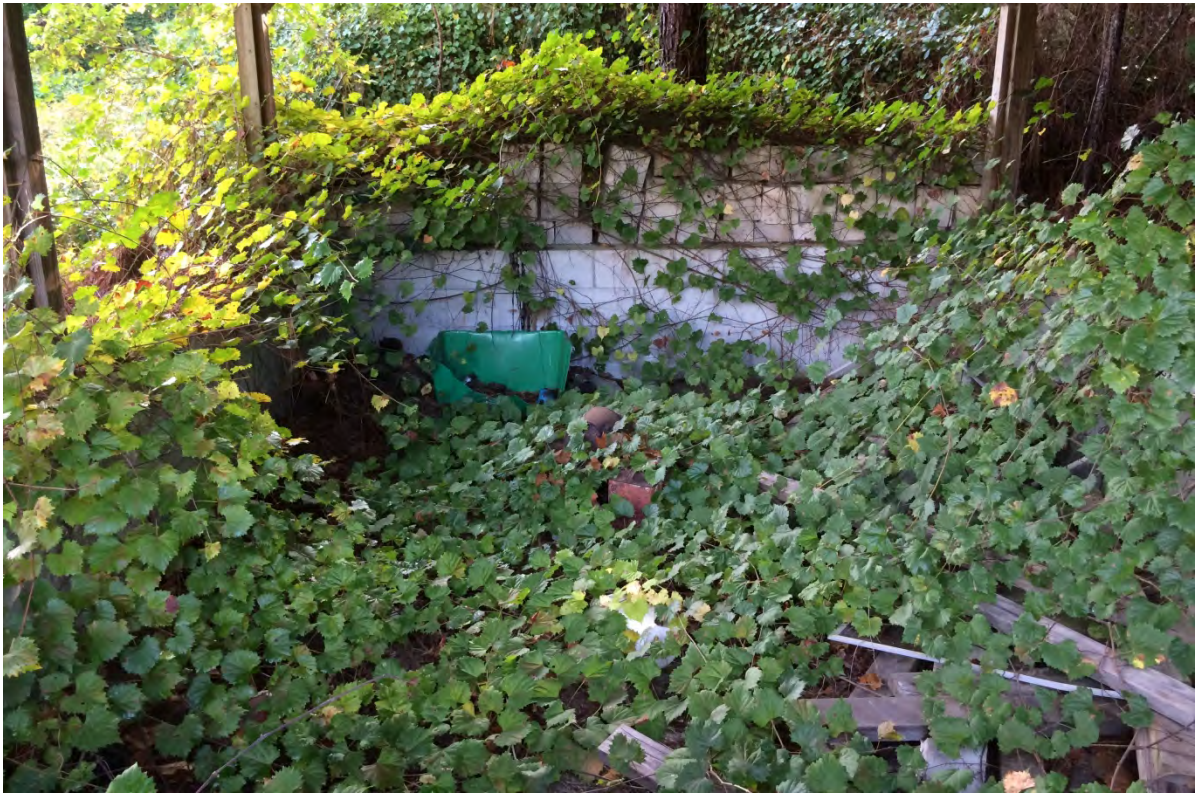
Site 110: The Pines Golf Club and Maintenance Facility – rusted containers in pavilion
