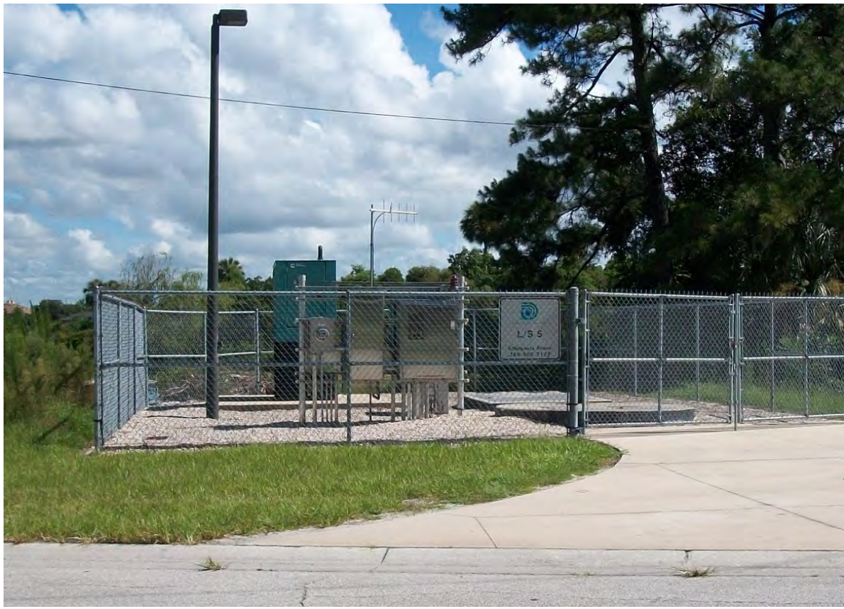
Site 13: Deltona LS #5 Generator
