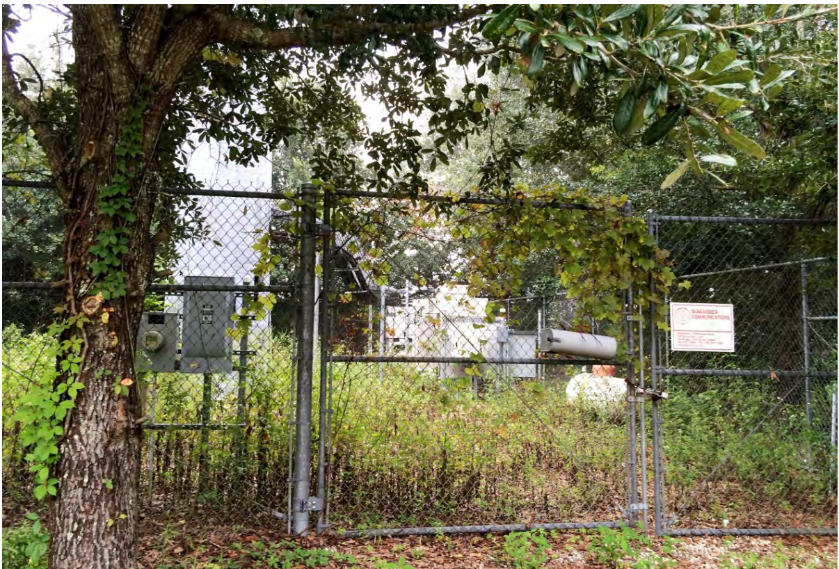
Site 108: Cell Tower with Diesel Powered Generator
