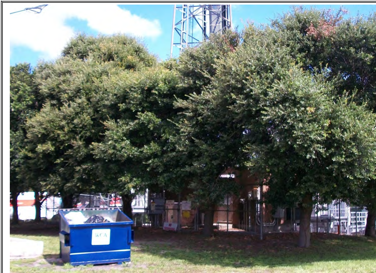
Site 76: Cell Tower with Diesel Generator
