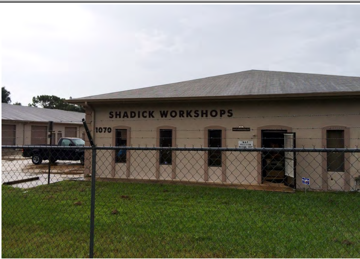
Site 119: Multiple Businesses located at 1070 Shadick Drive
